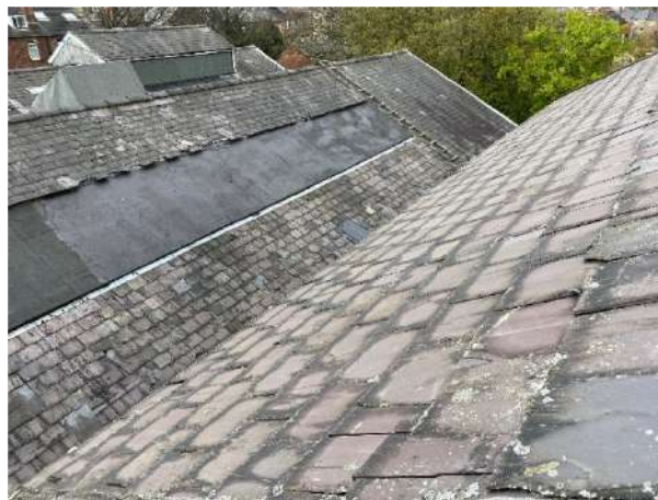
Figure 5 - Life expired slate roof coverings
