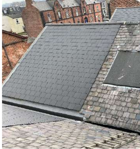
Figure 4 - 5m of overlaid roof to eastern end of pitched roof
