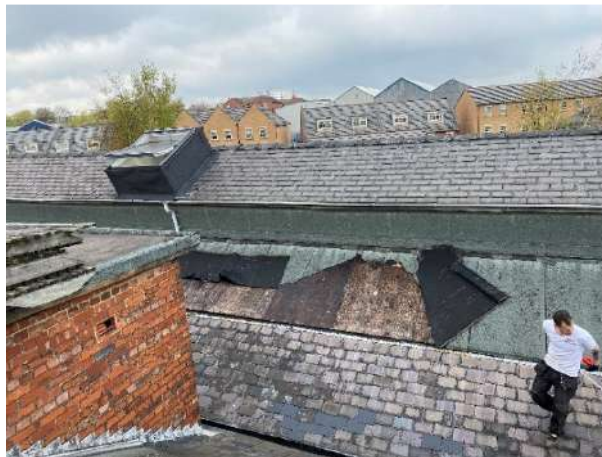
Figure 7 - Exposed plywood infill to previous roof windows
