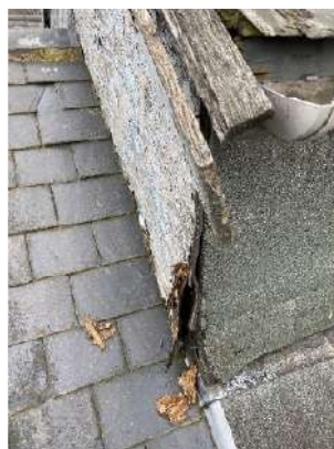
Figure 8 - Weathered timber finishes to monitor (E)
