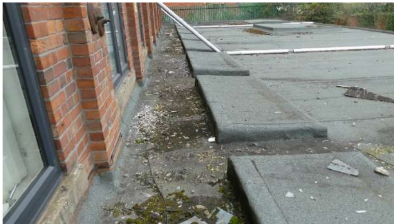
Figure 9 - Upstands to flat roof over single storey extension
