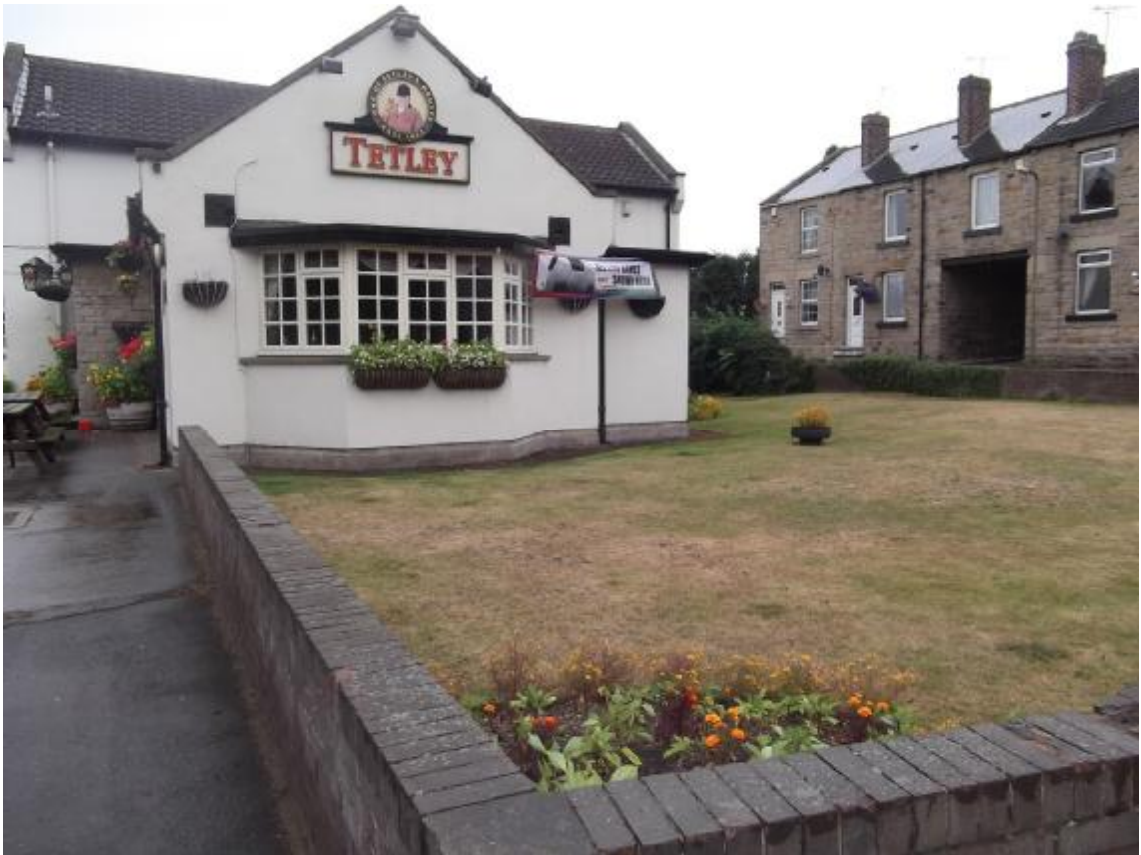
Fig 3: - Photograph showing the front of the premises & boundary wall and beer garden.
