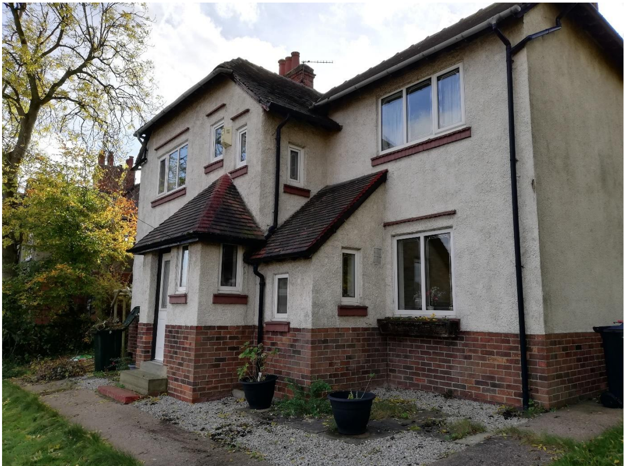
Photo 1. External elevations. Front elevation, right side.
