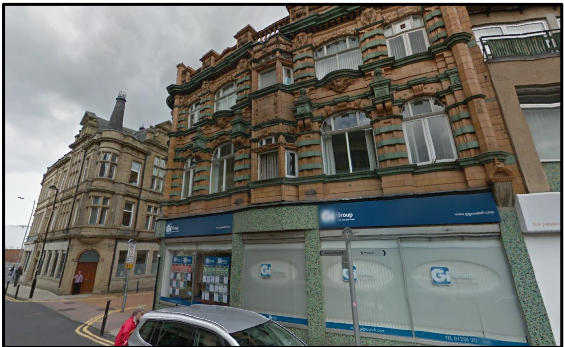
Fig.8. Image of listed buildings opposite the site
