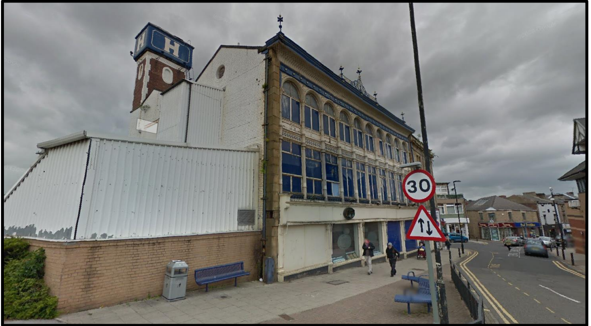
Fig.6. Former listed building on site fronting New Street
