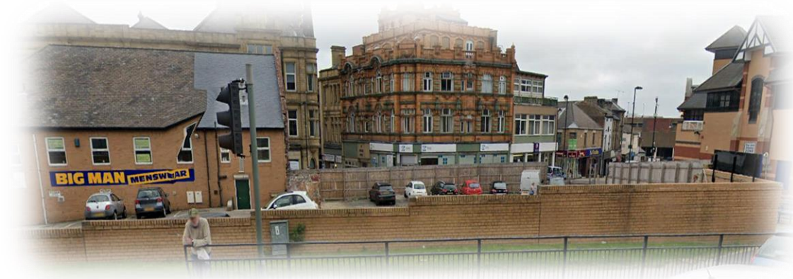
Fig. 3: View of site from West Way, showing the corner of Francis Jordan House to the west with the entrances to New Street and Market Street beyond.
