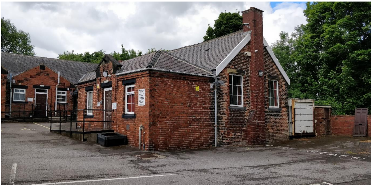
Existing Site Photo
