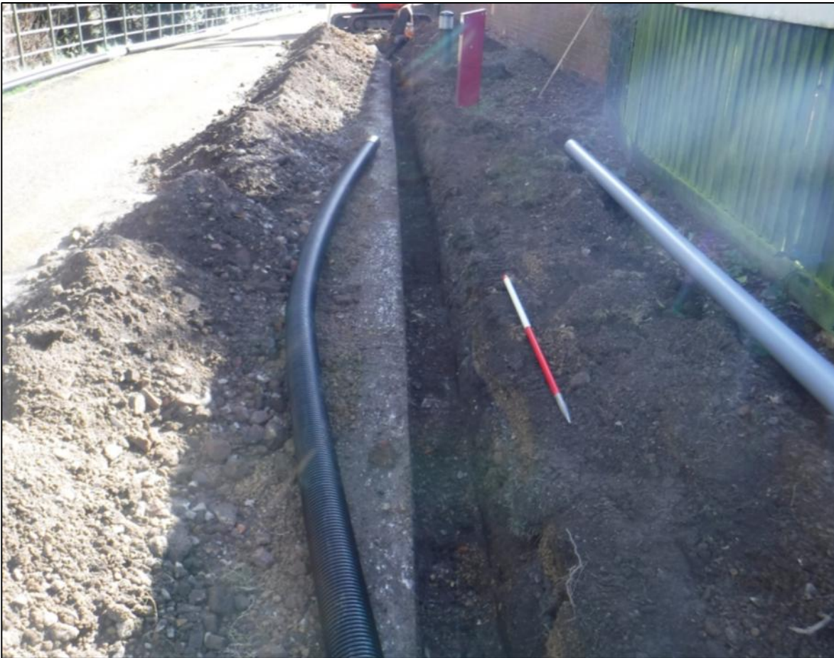
Plate 3. Trench 2, looking southeast.
