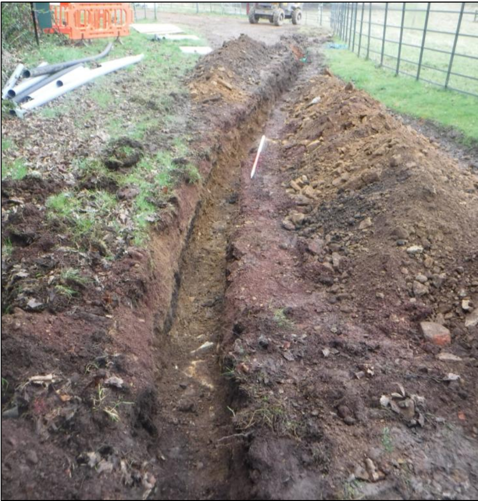
Plate 7. Trench 6, looking northeast.
