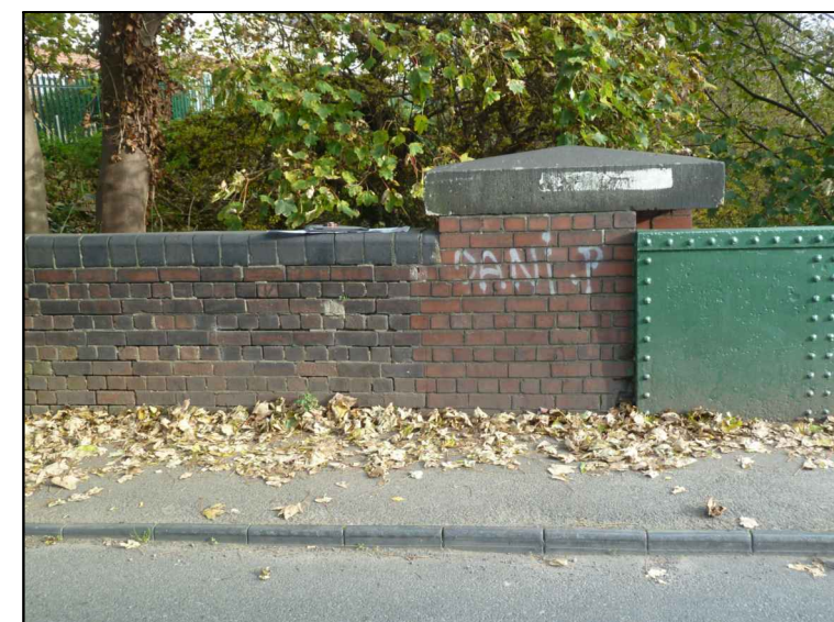
VIEW 6 EAST SIDE PARAPET
