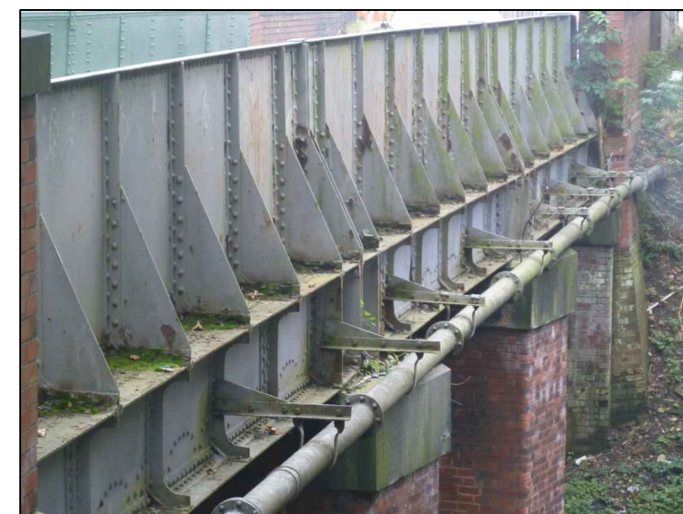
VIEW 5 REAR VIEW OF WEST SIDE PARAPET
