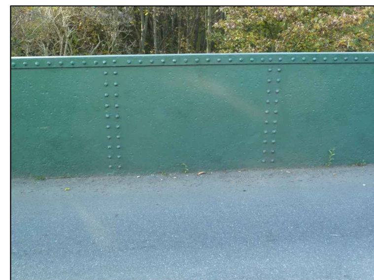
VIEW 3 WEST SIDE PARAPET
