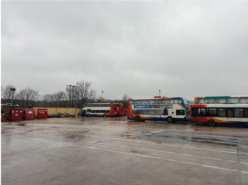
Figure 5. View of the developed land, sealed surface on site (February 2026).
