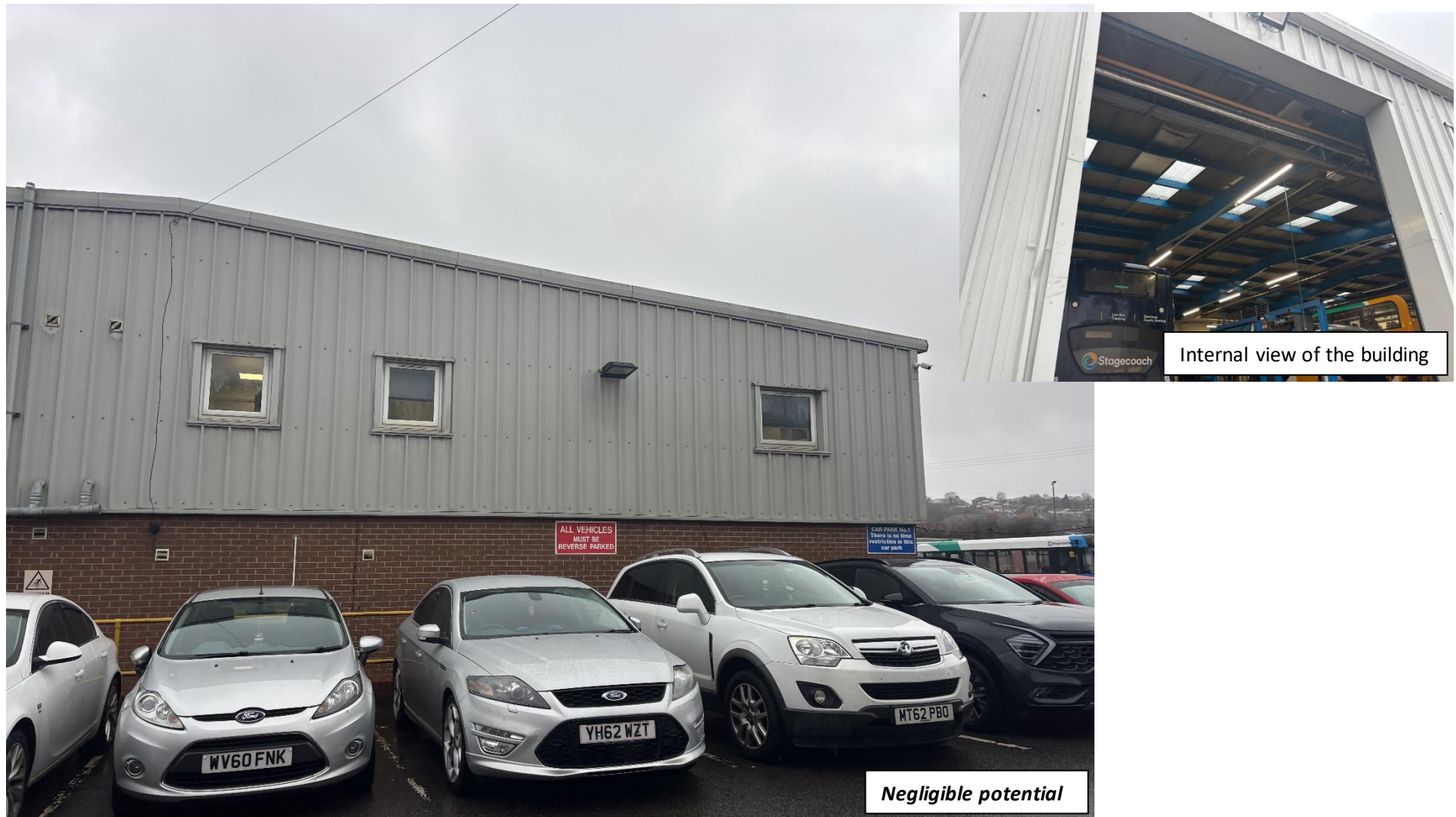
Figure 7. Bus Depot and servicing building with negligible bat potential (February 2026).
