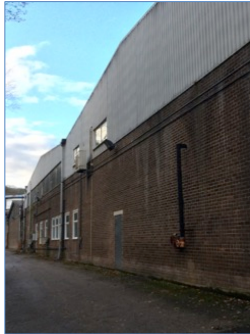
Photograph 41. External view of B2I (TN8), viewed facing west
