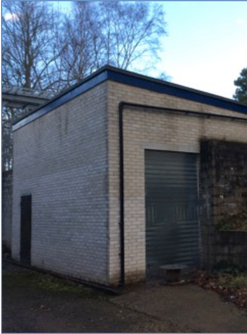
Photograph 28. Typical brick and flat roof construction – B28
