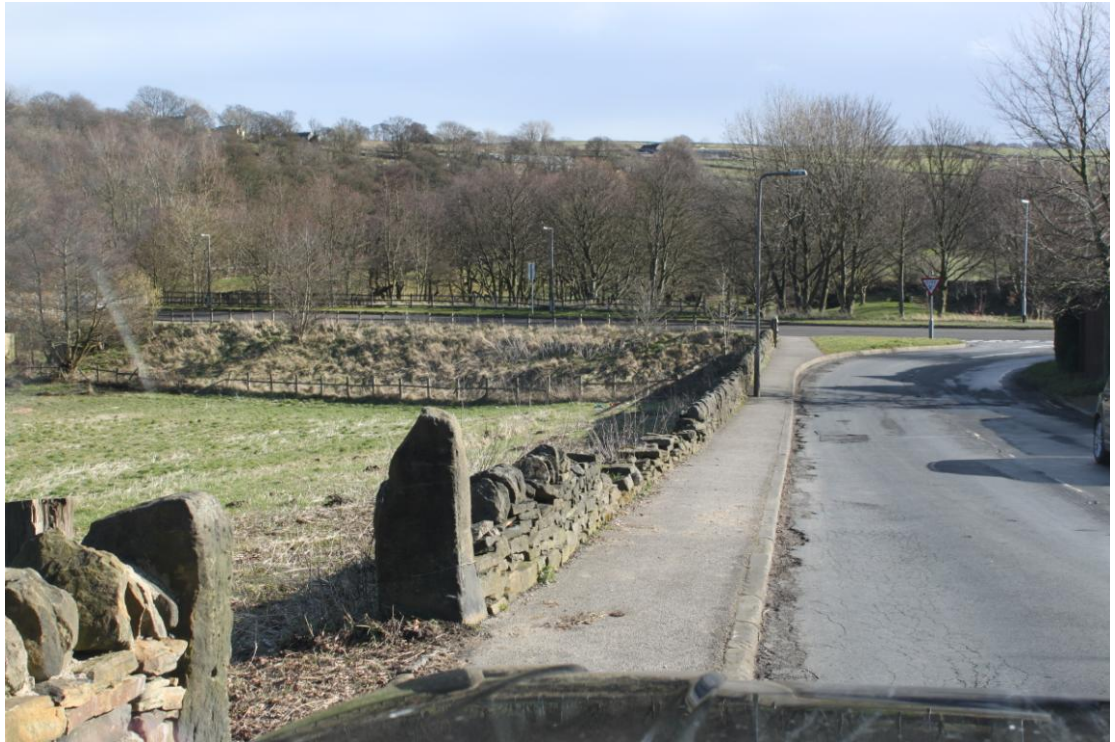
PADDOCK SITE ROUGH BIRCHWORTH LANE , OXSPRING – EXISTING SITE ACCESS
