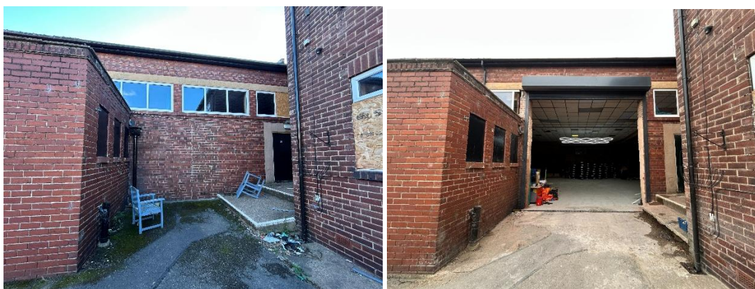
Image 3.1: Installed Roller Shutter
