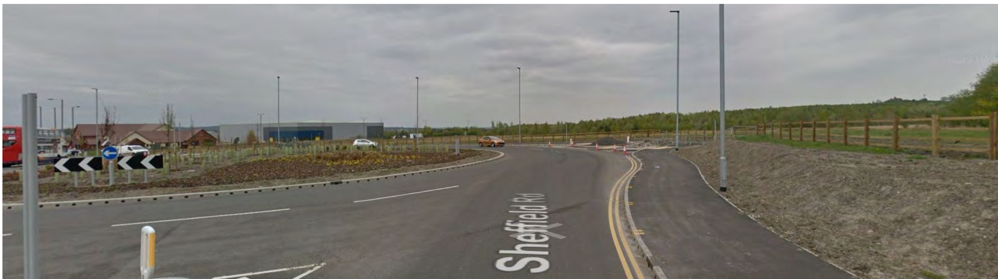
Street View looking West From Sheffield Road
