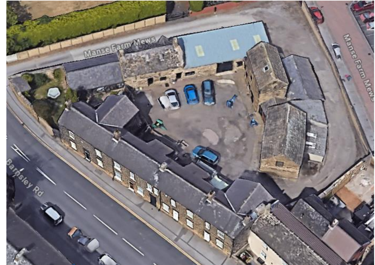
Figure 1 Overview of Manse Farm (Source: Google Maps).
