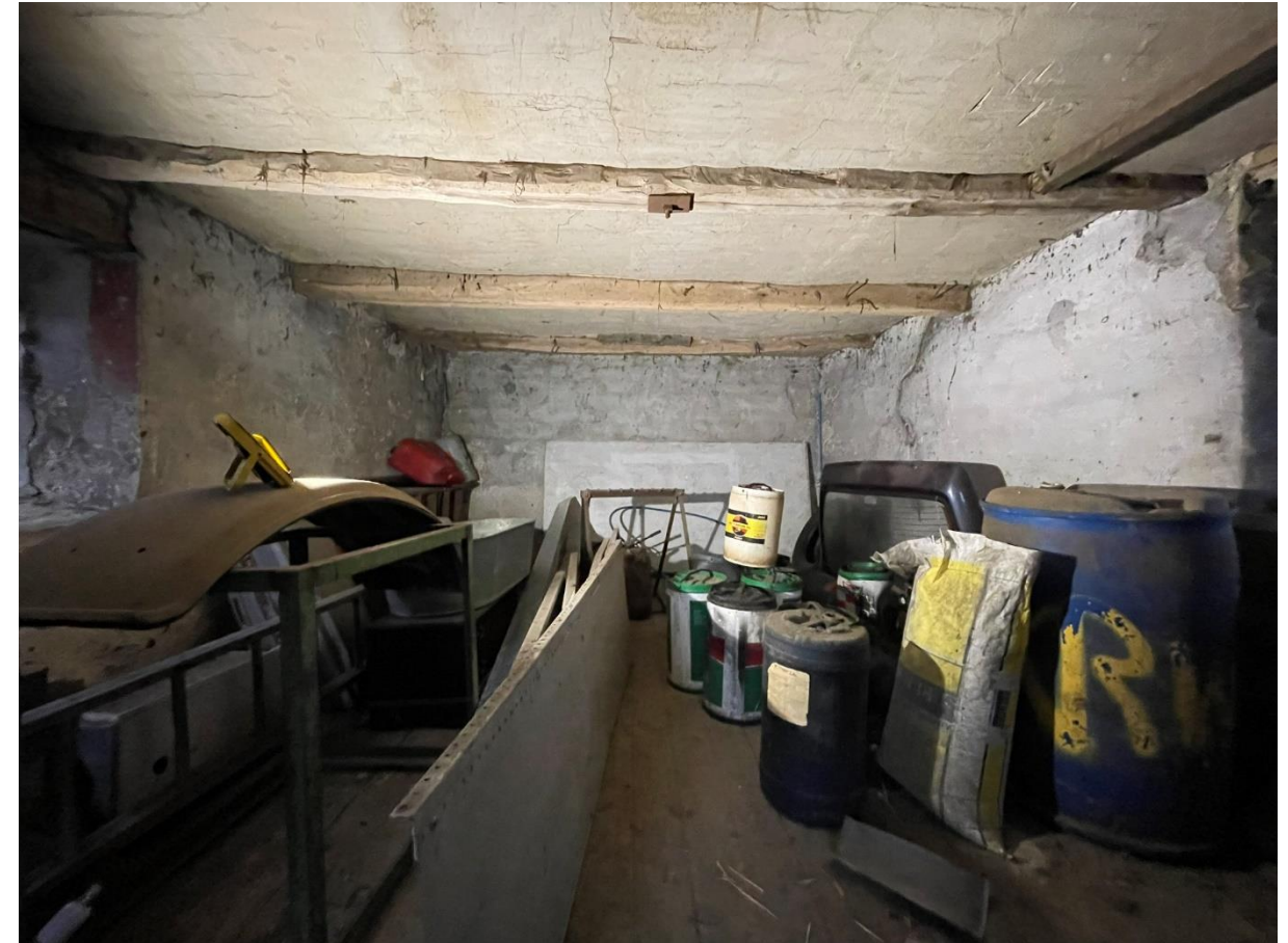
Figure 24 View of underside of second floor in main building.
