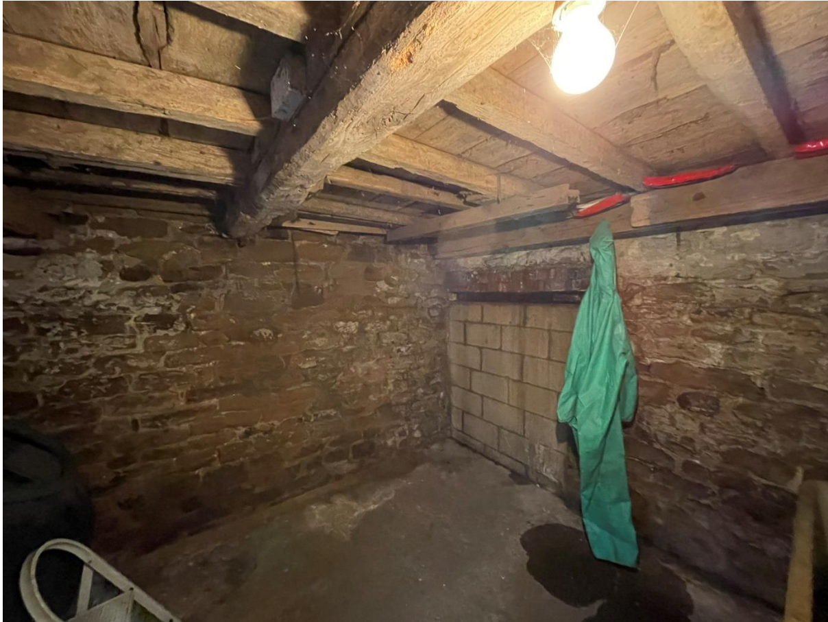
Figure 23 View of underside of first floor in main building.
