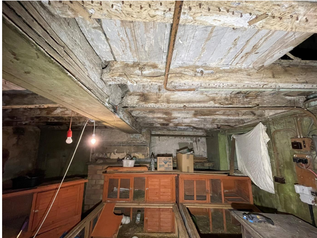
Figure 14 View of the underside of the first floor.
