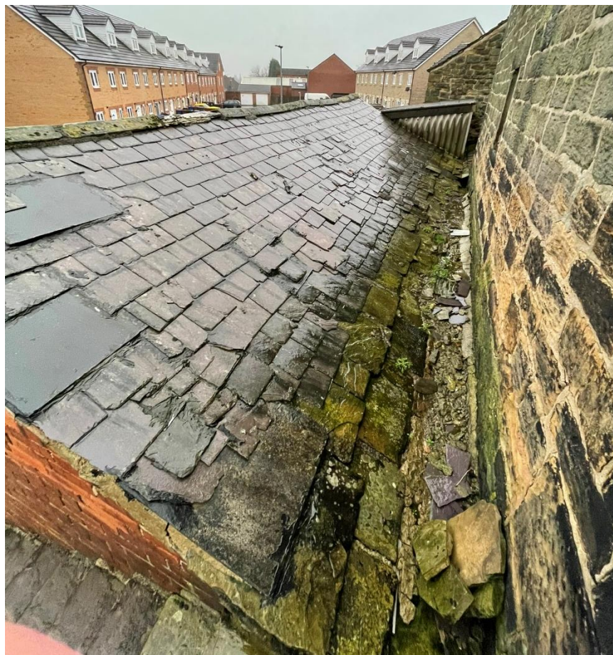
Figure 21 Valley gutter of covered area against main building.
