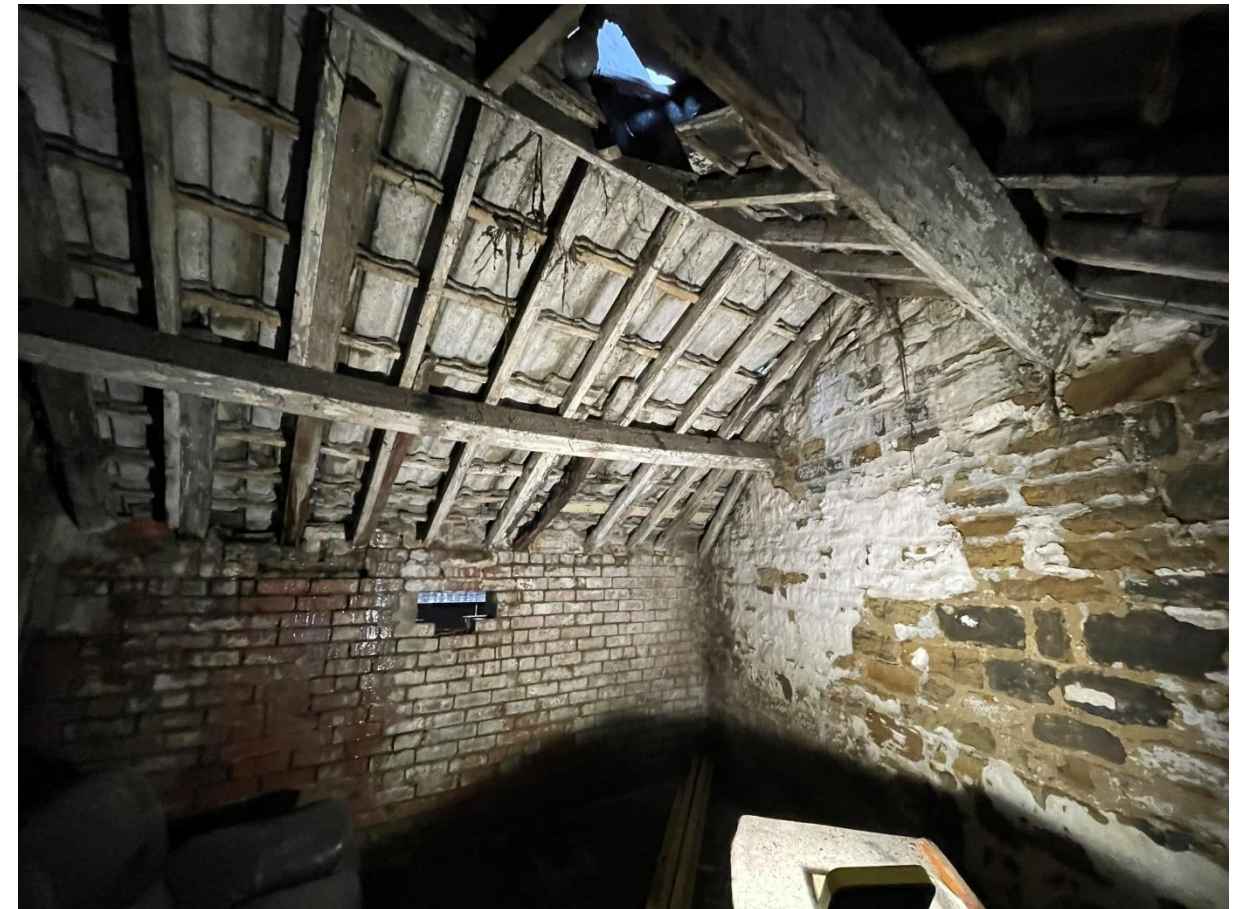
Figure 22 View of roof structure in The Stable.
