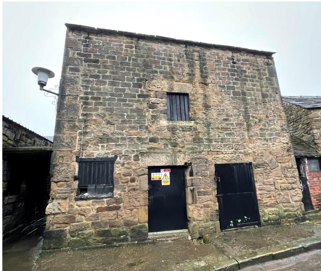
Figure 15 West elevation of main building. Partially infilled first floor window visible.
