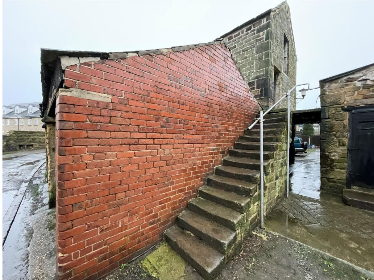
Figure 17 Brick wall to north elevation of covered area.
