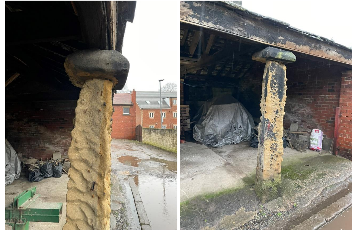
Figure 18 Stone columns to east elevation of covered area.
