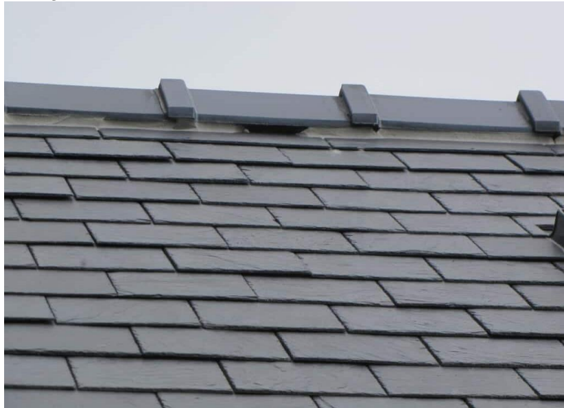
Figure 4. Example of bat access point in the ridge
