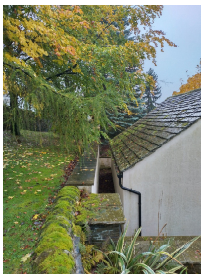
Photo 4: T5 and T7 from east - western crowns extending over roof
