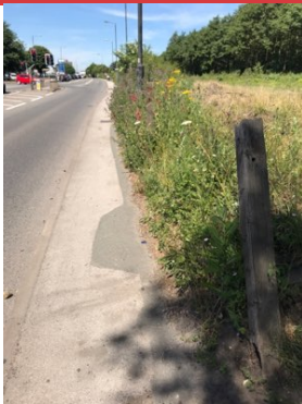
ISSUE 31 DAMAGED FENCE ADJACENT TO TESCO BELL MOUTH
