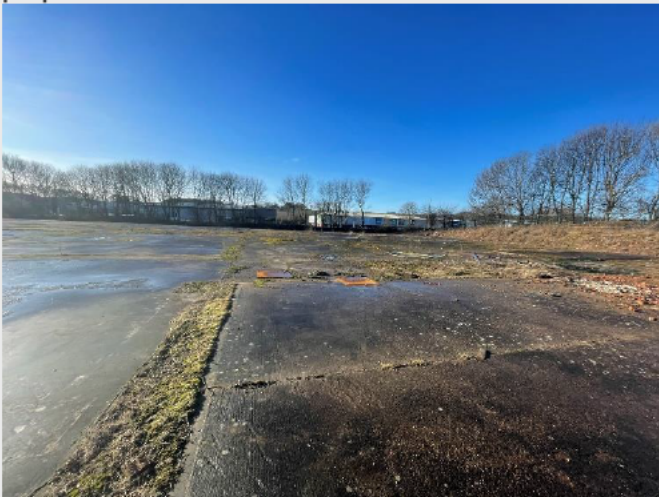
Photograph 7: Hardstanding at western extent of site
