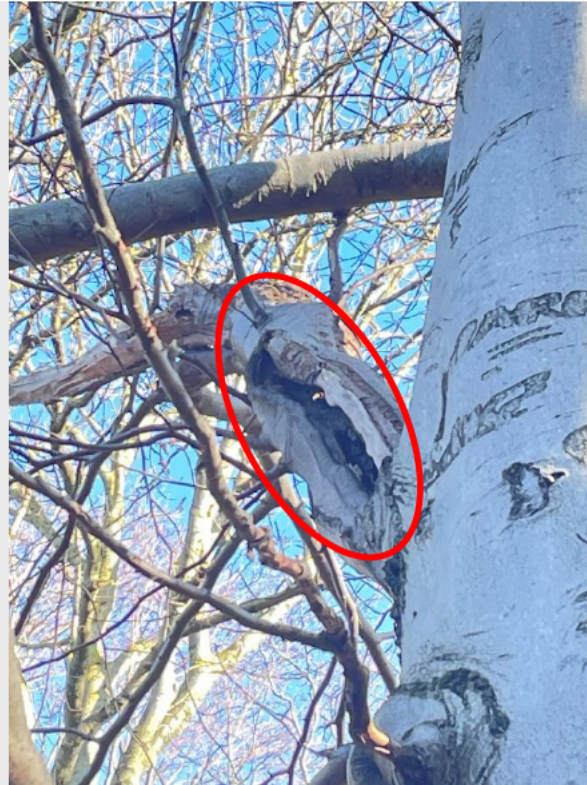
Photograph 14: T1 - PRF-A, hazard beam
