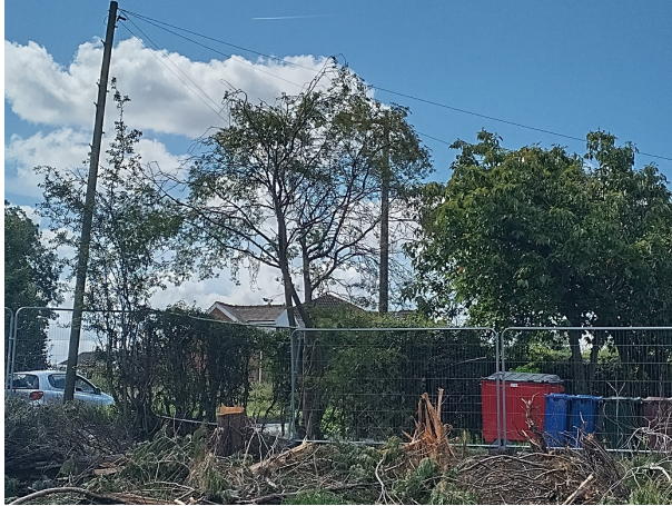
Photo 1: T1 looking south
