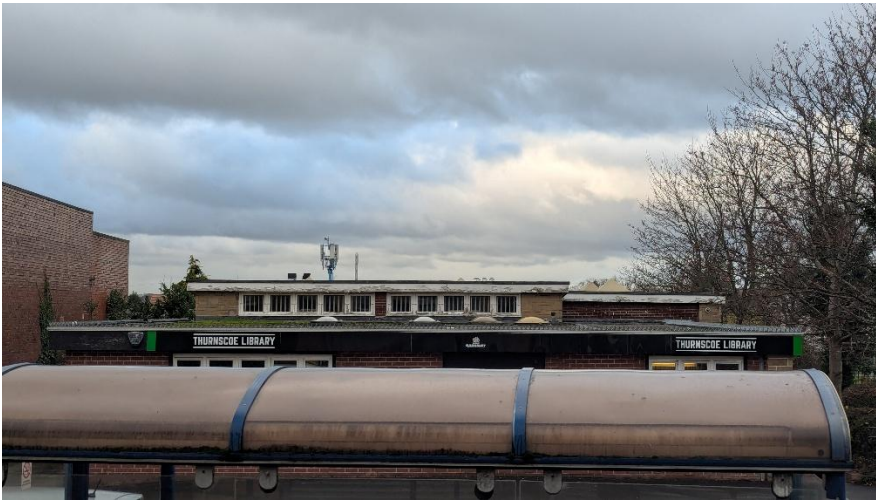
Figure 6 View of the roof from the south over the road.
