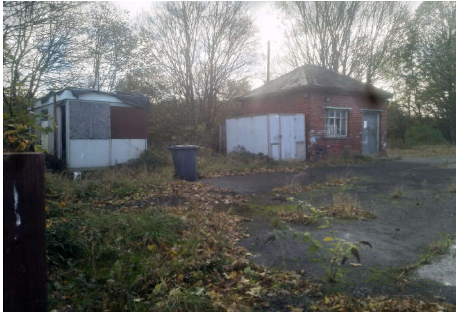
Brick building and portacabin
