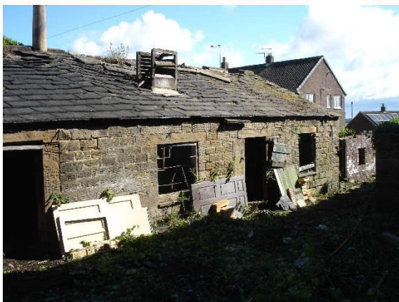
Fig 07. Stone Outbuilding to rear.
