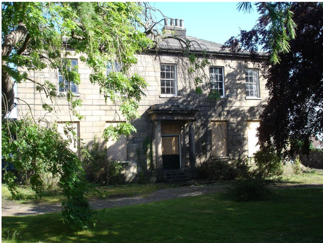
Fig 01. Front [South] Elevation of Osborne House
