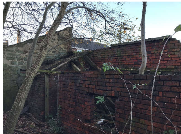
Fig 08. Brick Outbuilding to rear.
