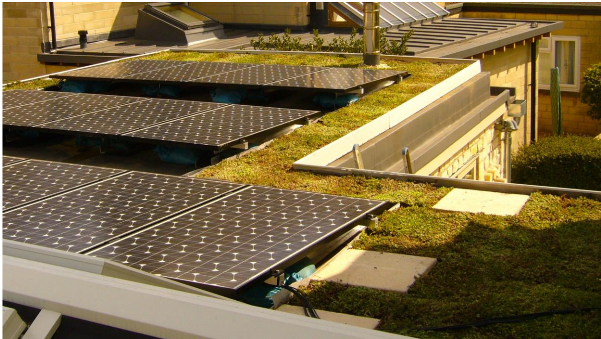
Example of green sedum roof with solar panels
