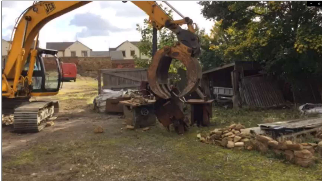
Plate 1. A photo of the site taken during the demolition of the barn in 2019 showing ephemeral vegetation on hardcore across most of the site
