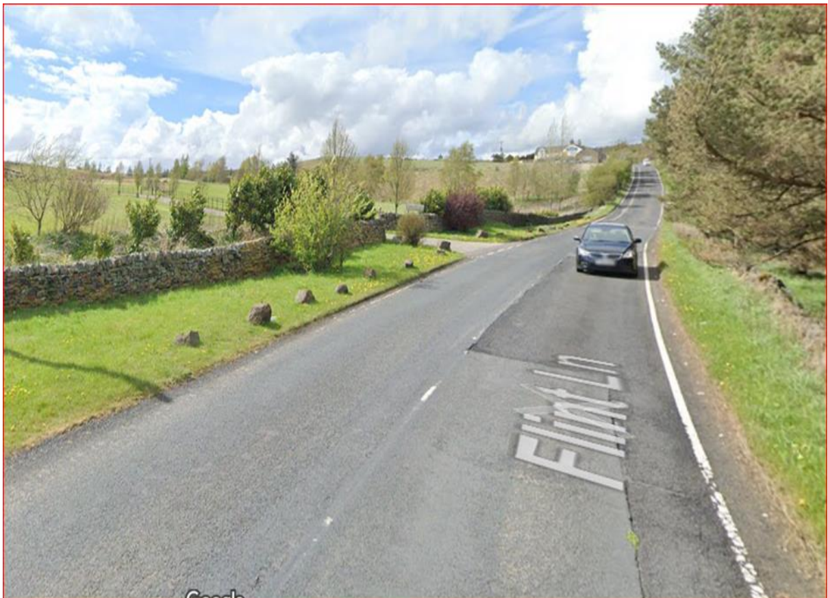
View of access onto the highway, looking north-west.
