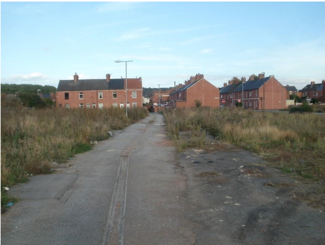
Photograph 08: view east along Main Street from Central Street
