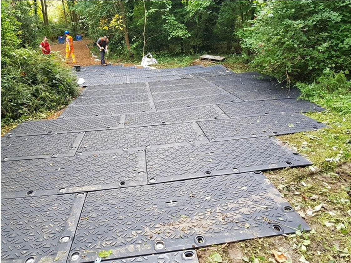
Figure 6: Interlinked ground protection boards placed on top woodchip
