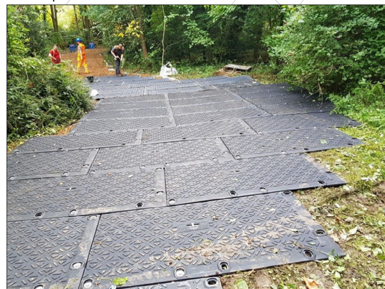
Ground protection boards
