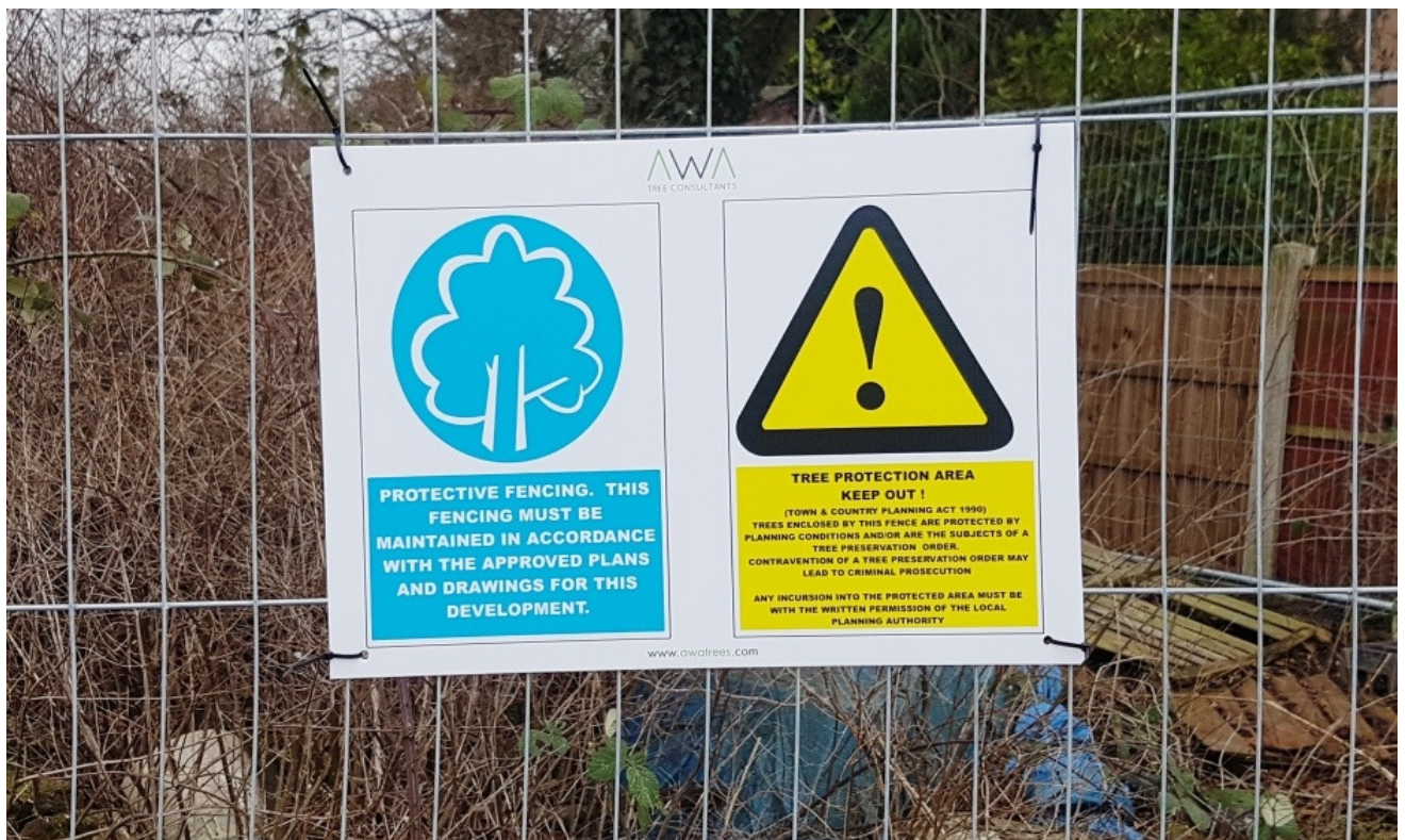
Figure 5: Example of A3 correx tree protection warning sign fixed to fencing panel
