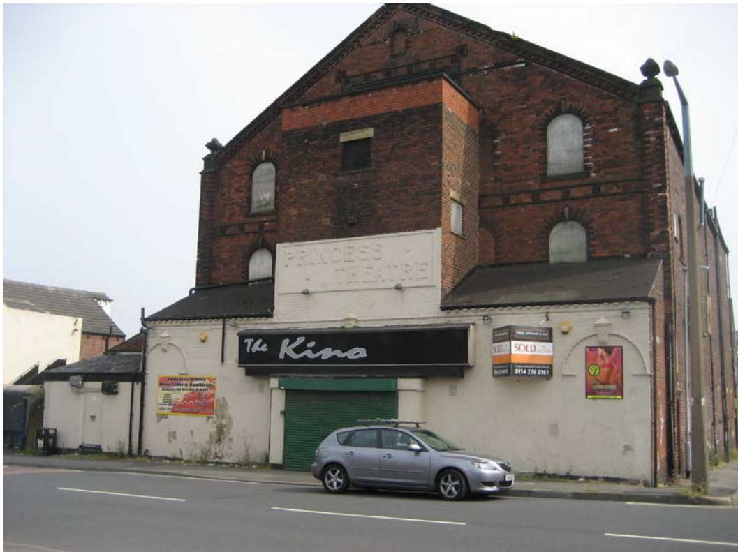
View of the existing building from the North.
