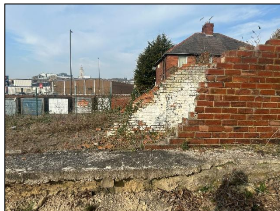
Figure 3.2: Hardstanding to north of site.
