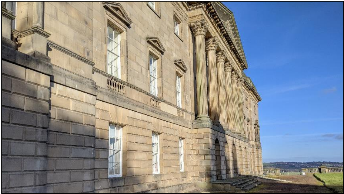
Figure 2. Crevices in south elevation masonry, visible from ground, which are considered to display bat roost potential
