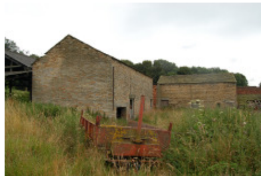
The Barns from the Entry Road
