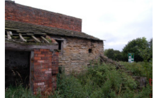
Lean too, to be demolished and rebuilt in stone
