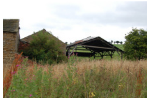
Lean too, to be demolished and rebuilt in stone
