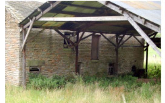
Dutch barn demolished, lean too built on end gable to replace
