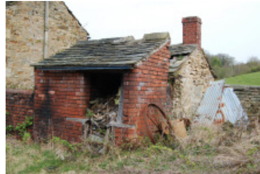
Free standing building demolished and rebuilt in stone as a garage
