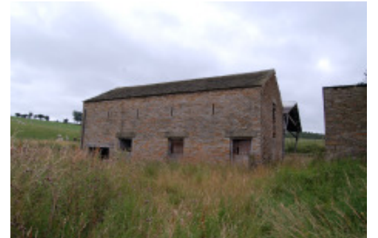
Barn A From Courtyard
