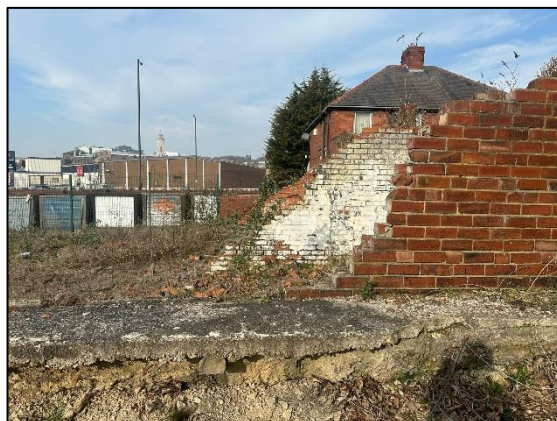
Figure 3.2: Hardstanding to north of site.
