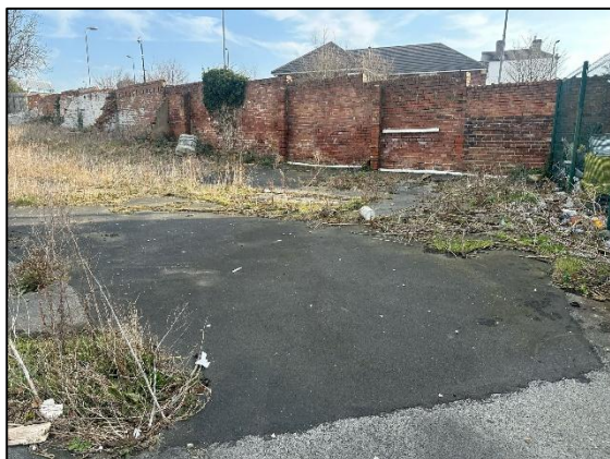
Figure 3.1: Hardstanding to south of site.
