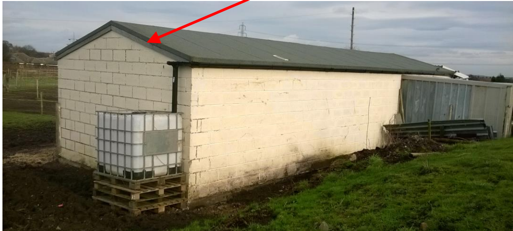
Plate 3 West gable and south elevation. Barge board
