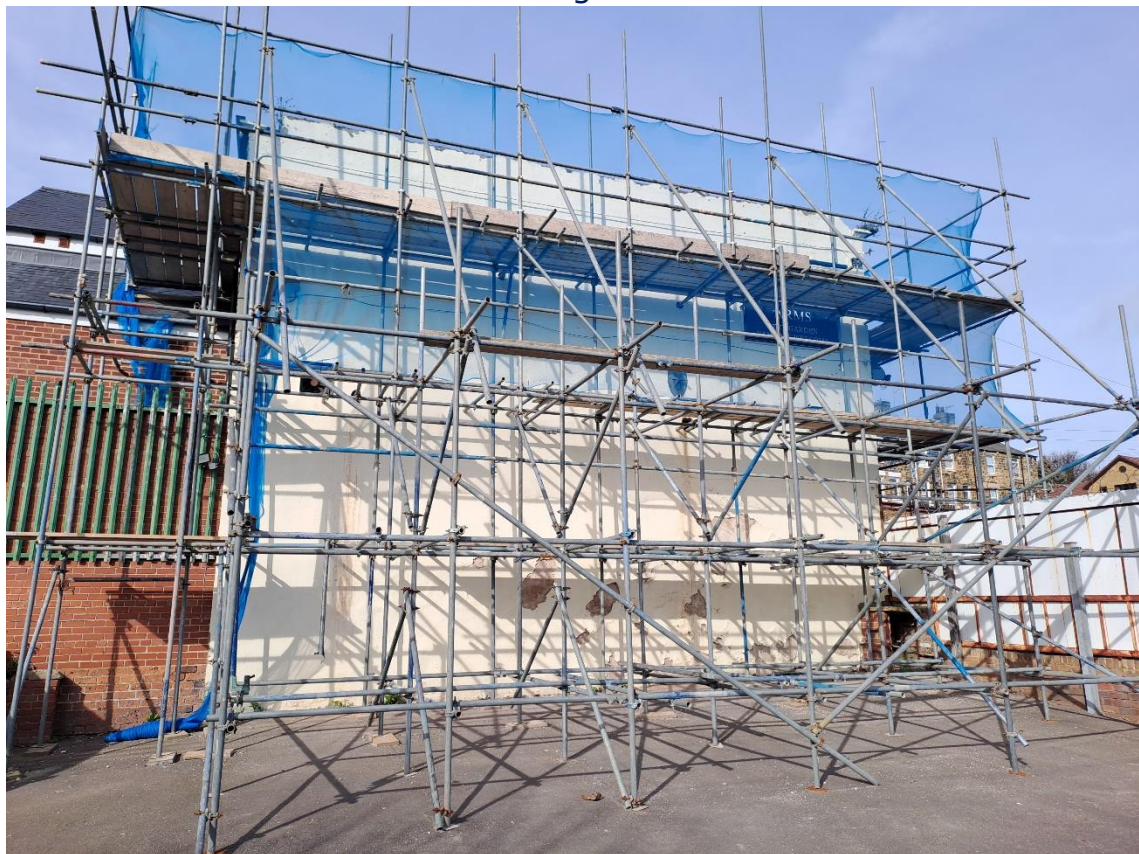
Side Elevation showing the scaffold bracing.
