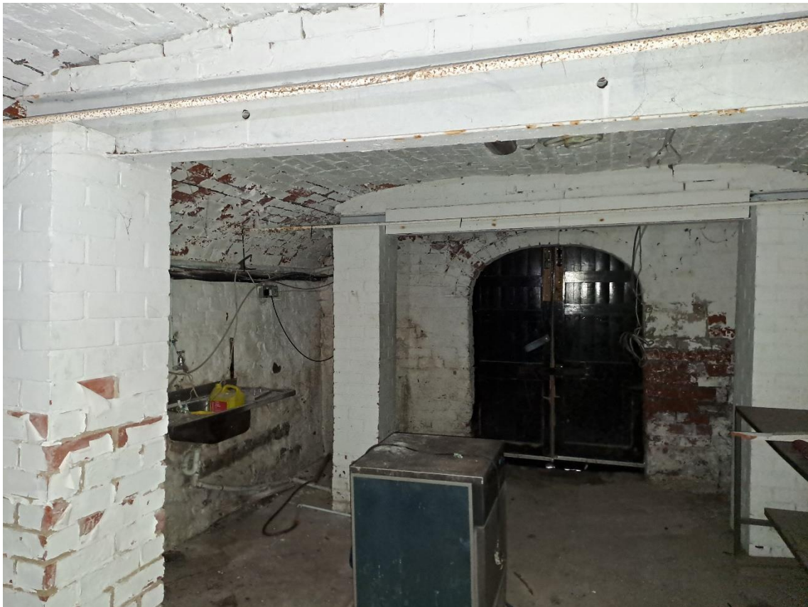
Basement view showing the flattened arch and steel support beam.
