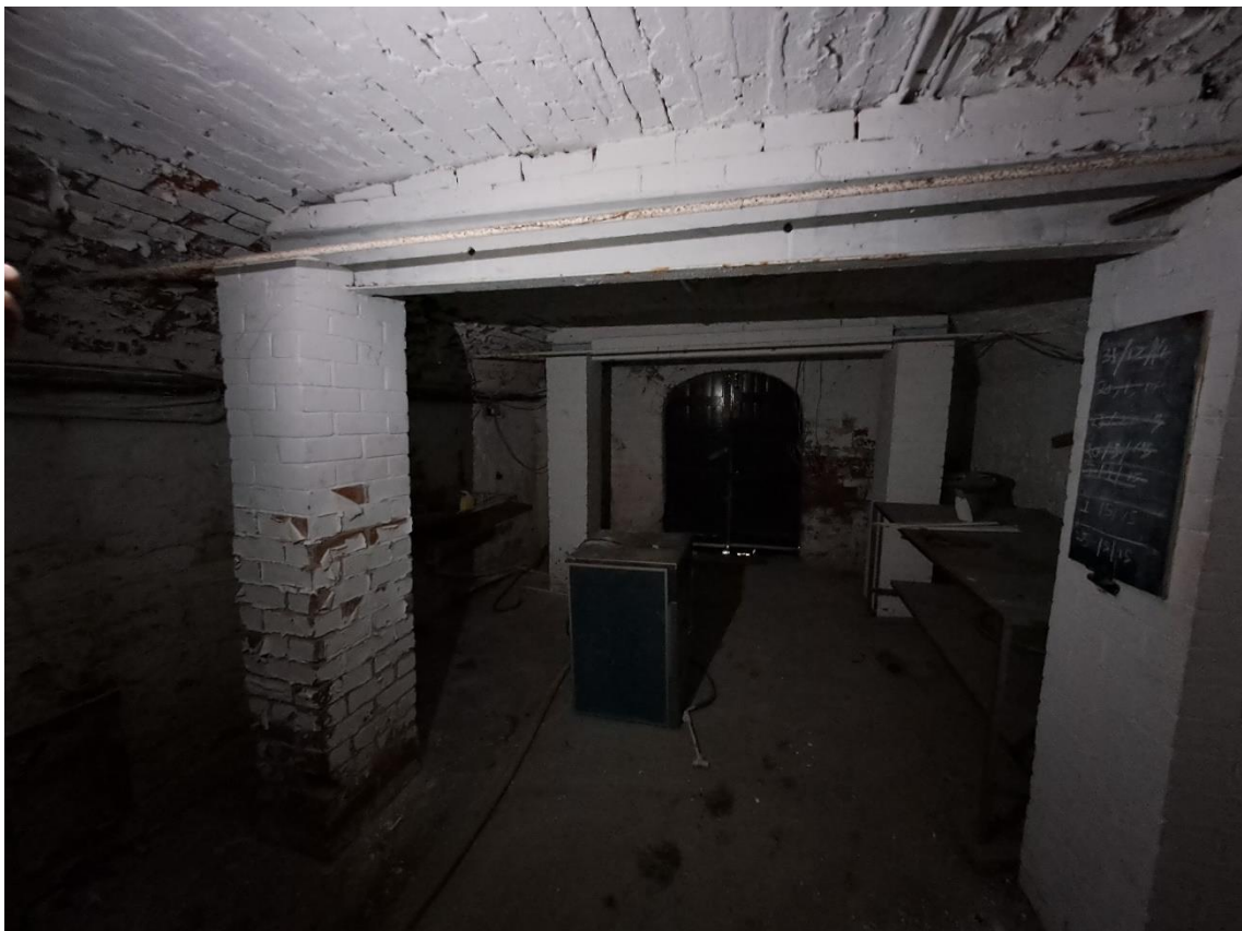
Basement view showing the flattened arch.
