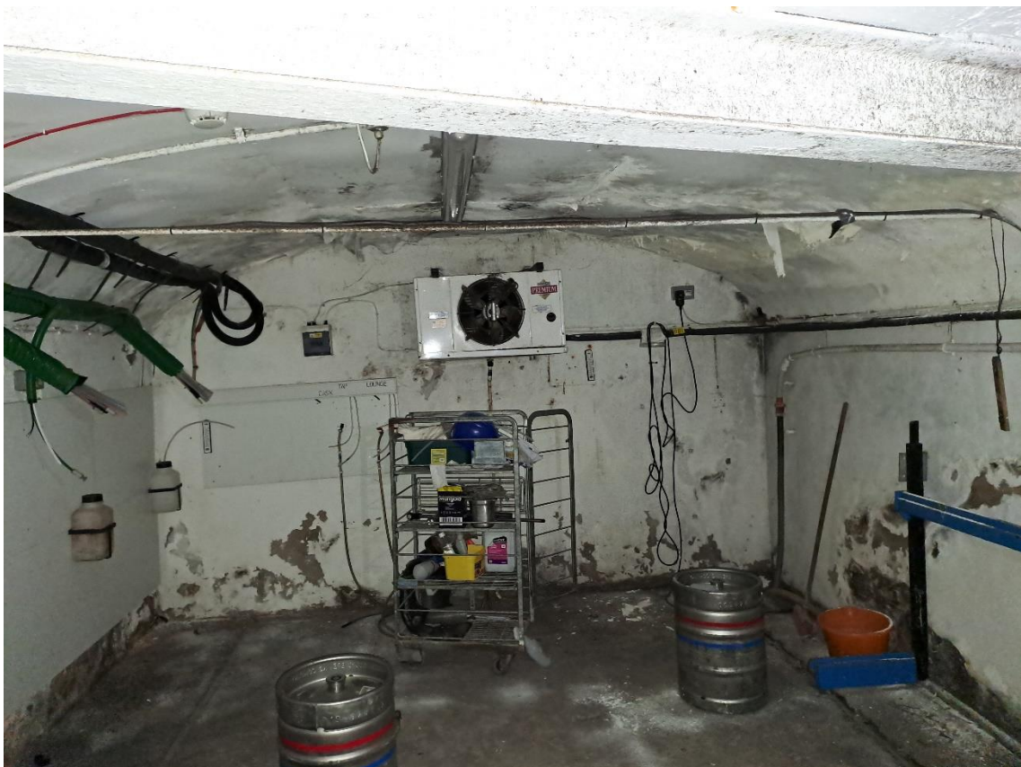
Basement view showing the steel support beam.
