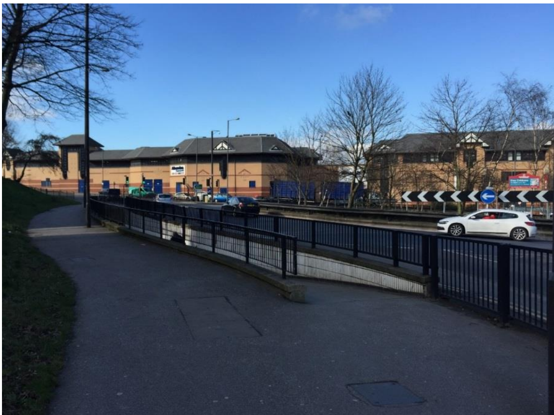
Photograph 3 Pedestrian subway at the Alhambra Roundabout
