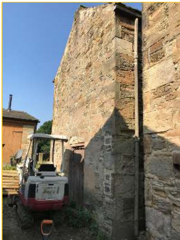
Photograph - 15 - Right extension rear gable
