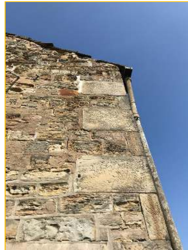
Photograph - 35 - Left extension
