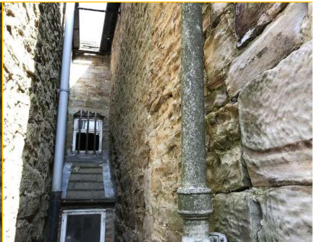
Photograph - 22 - Left extension
