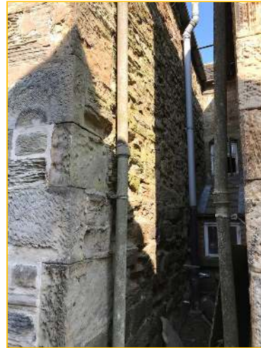
Photograph - 14 - Right extension left wall
