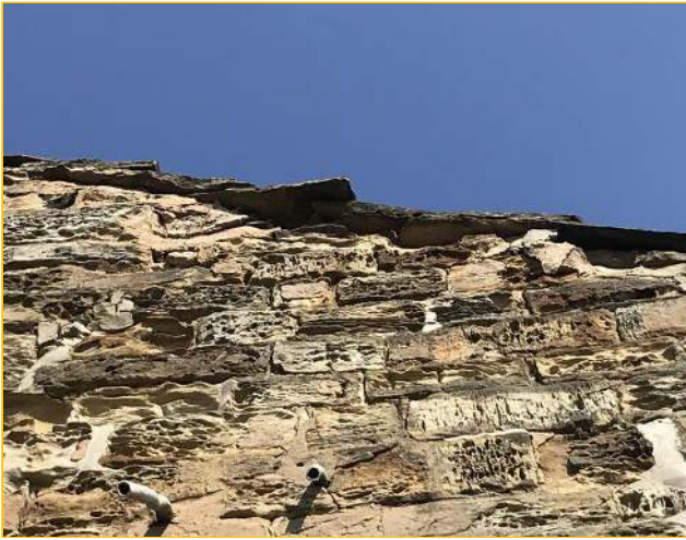
Photograph - 10 - Roof verge
