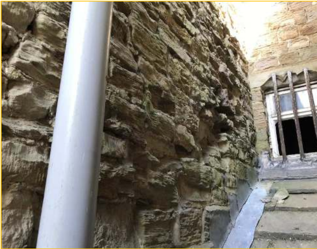
Photograph - 39 - Weathering
