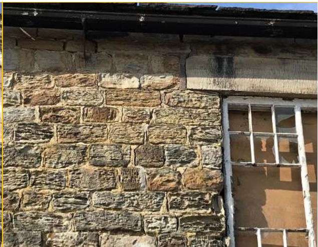
Photograph - 26 - Left extension
