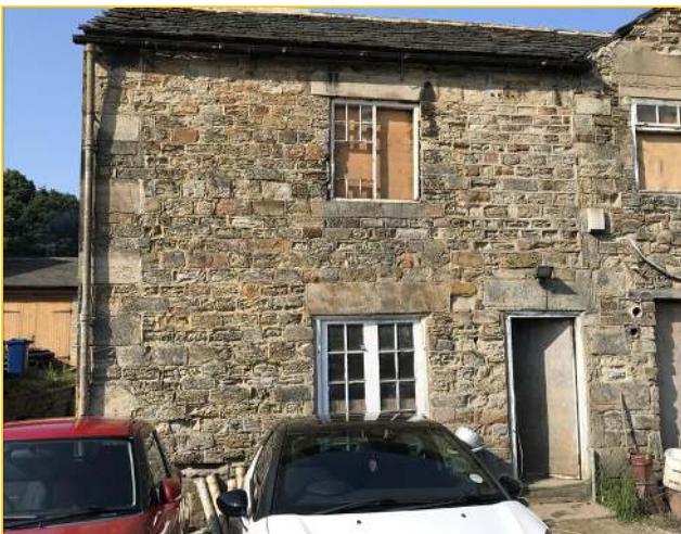
Photograph - 11 - Left extension left wall
