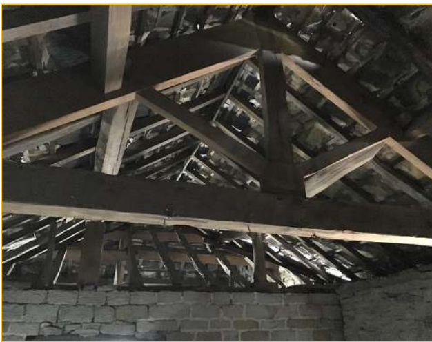
Photograph - 43 - Left hand extension roof
