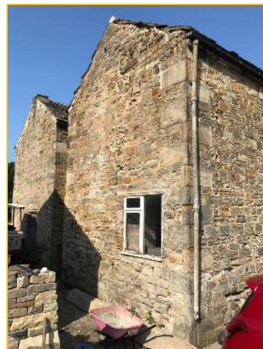
Photograph - 12 - Left extension rear gable
