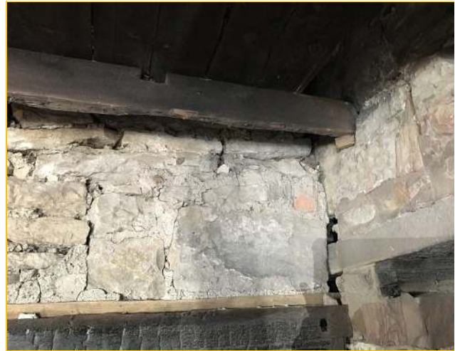
Photograph - 65 - Reflected fracture
