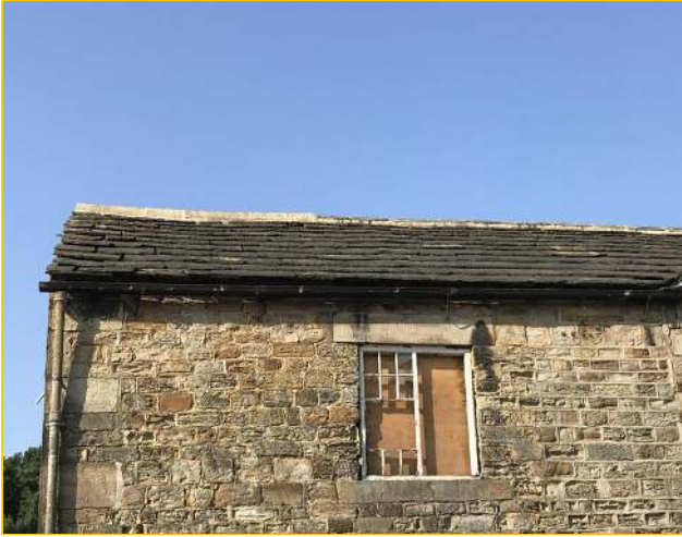
Photograph - 7 - Left hand slope
