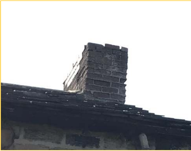
Photograph - 42 - Brickwork stack
