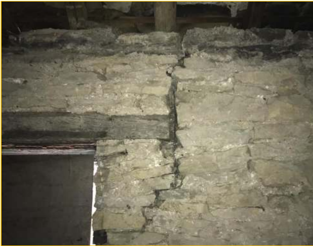
Photograph - 61 - Left extension
