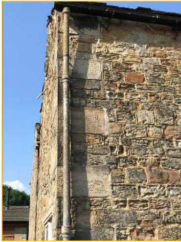
Photograph - 36 - Left extension
