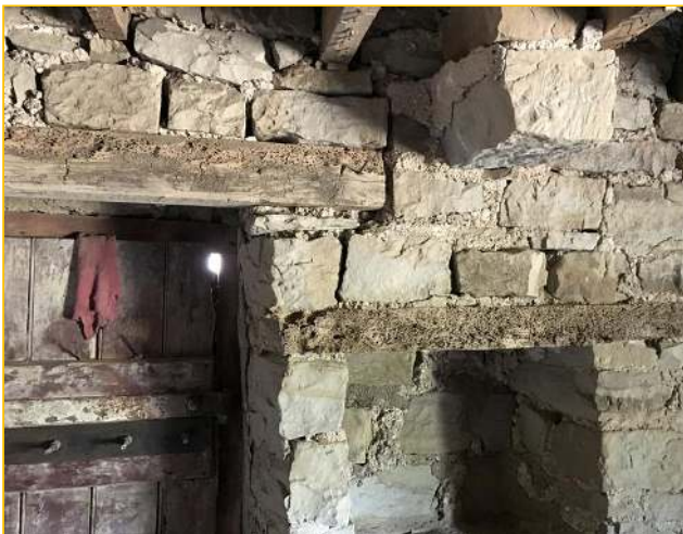
Photograph - 66 - Wood destroying insect damage
