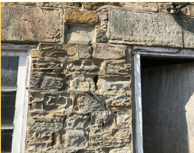
Photograph - 41 - Weathering
