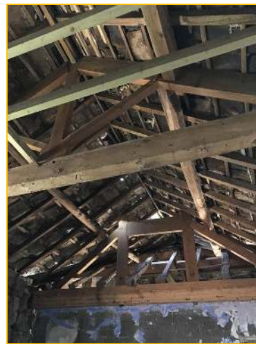
Photograph - 44 - Right hand extension roof
