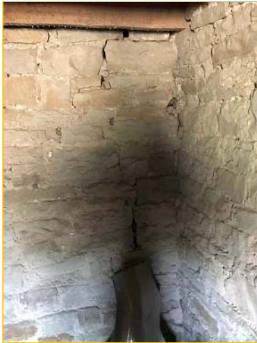
Photograph - 64 - Reflected fracture
