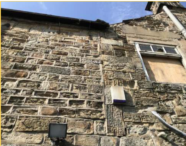
Photograph - 25 - Left extension
