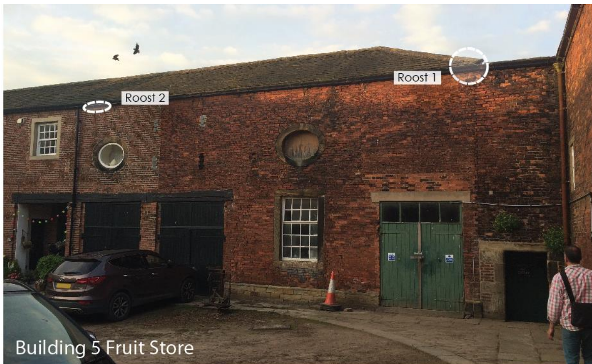
Figure 3 Western elevation of Building 5 - Roosts 1 & 2 highlighted
