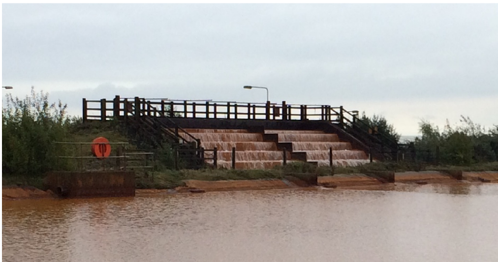
Figure 3 – Typical aeration cascade
