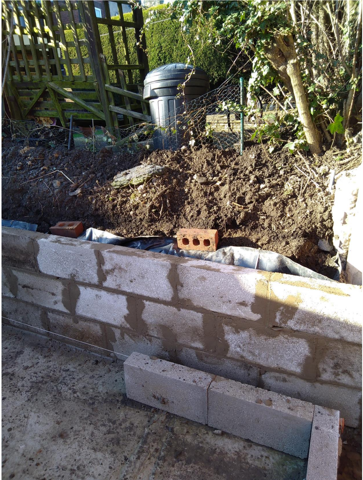
PHOTOGRAPH 10 SHOWS THE ONGOING WORKS TO THE EXTERNAL WALL OF THE BUILDING, ADJACENT TO THE EXISTING LAND, WITHIN THE CURTILAGE, WITH NO GAP. THE BLACK BIN THAT APPEARS IN MANY OF THE PHOTOS CAN CLEARLY BE SEEN.
