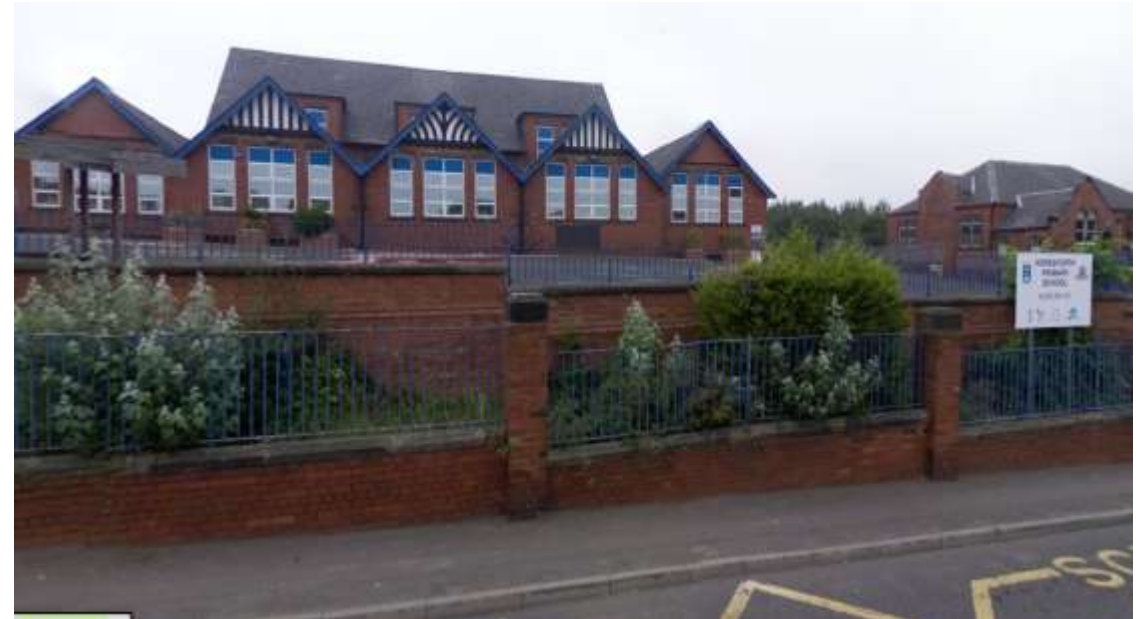
Fig 2.6: Keresforth Primary School
