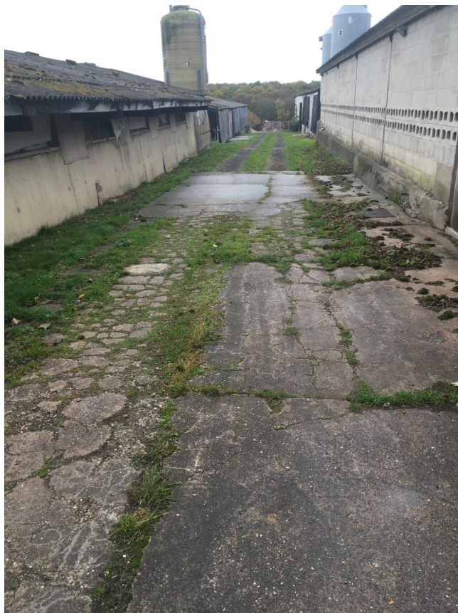
Looking south between the central and western row of sheds
