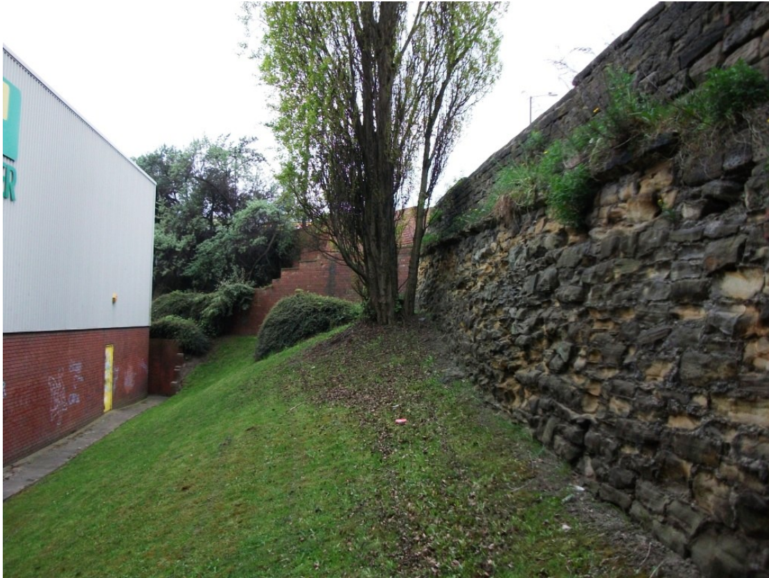
Plate 7: Retaining Wall, Showing Drop in Slope from Old Mill Lane
