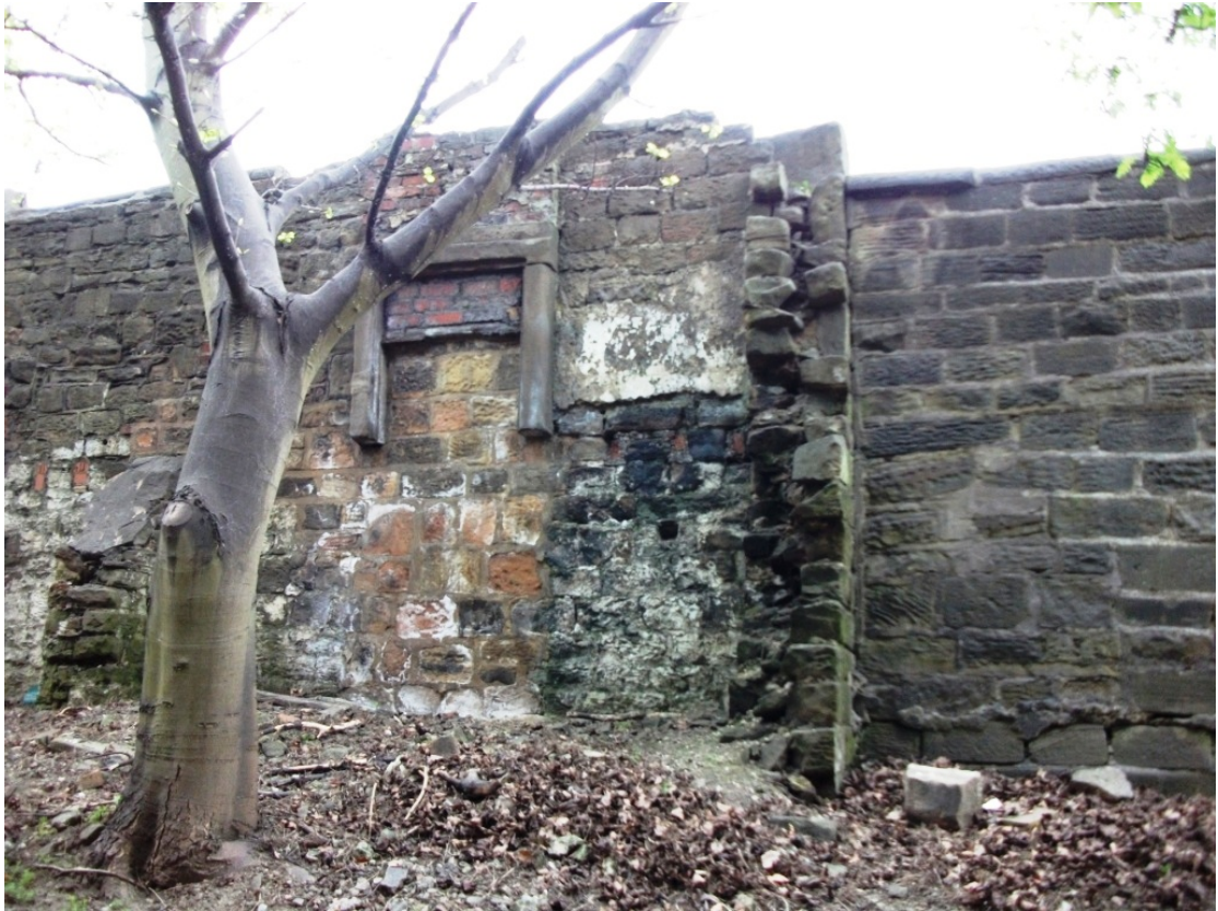
Plate 5: Elevated Hearth and Key-in Stonework on Western Retaining Wall
