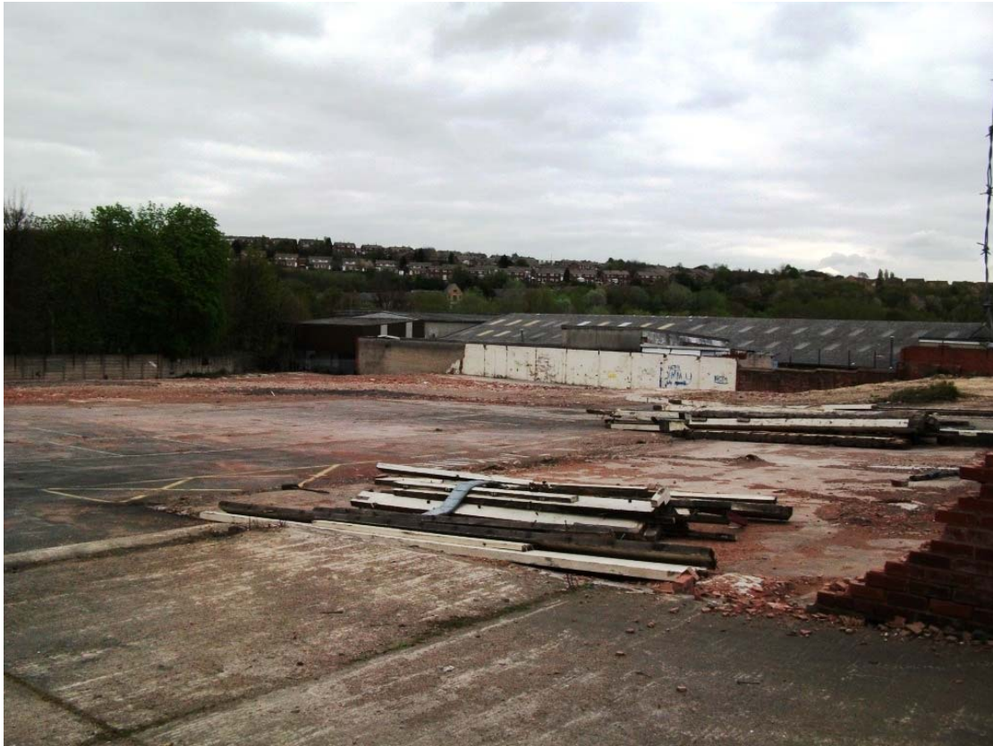
Plate 9: Area of Demolished Buildings, Looking Northeast from Twibell Street
