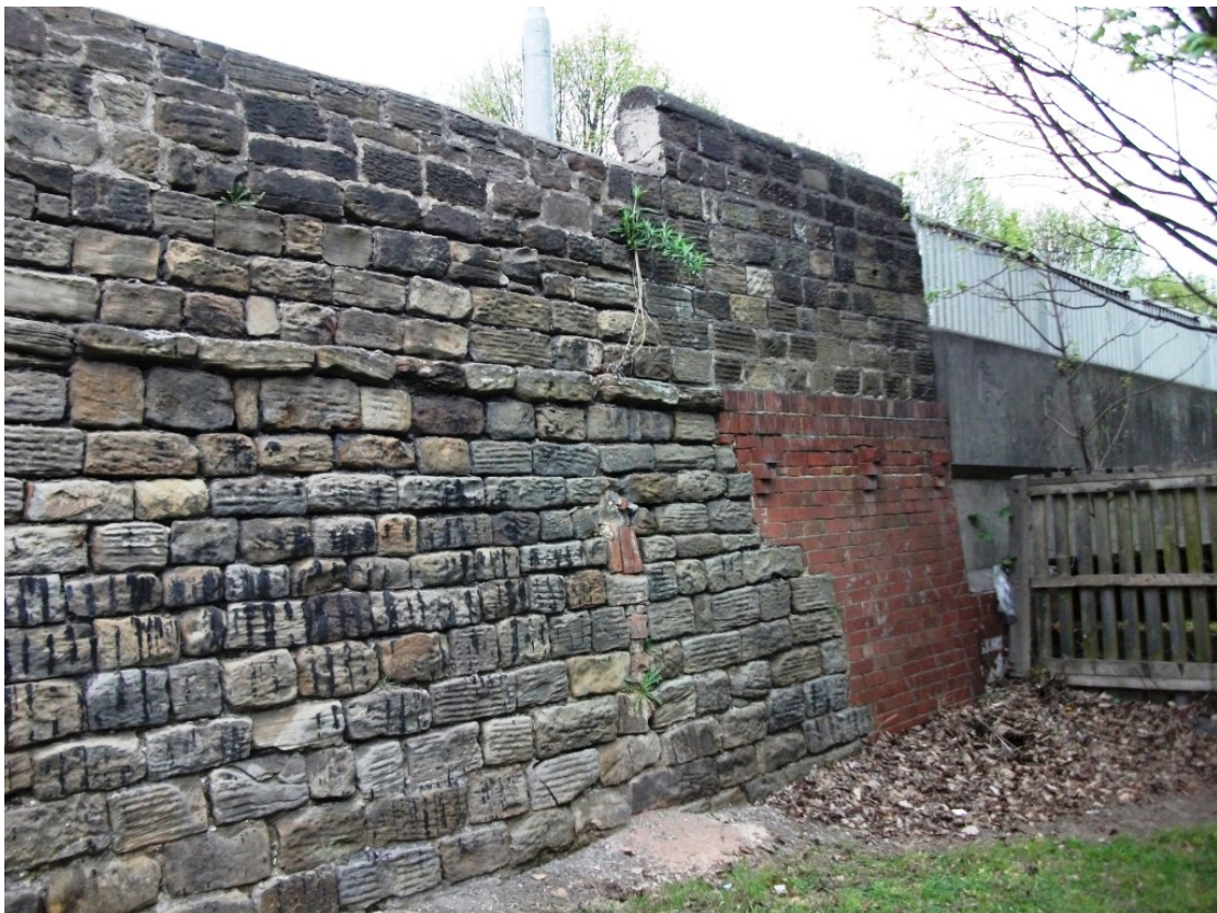
Plate 4: Retaining wall, just before the bridge over R. Dearne on Old Mill Lane
