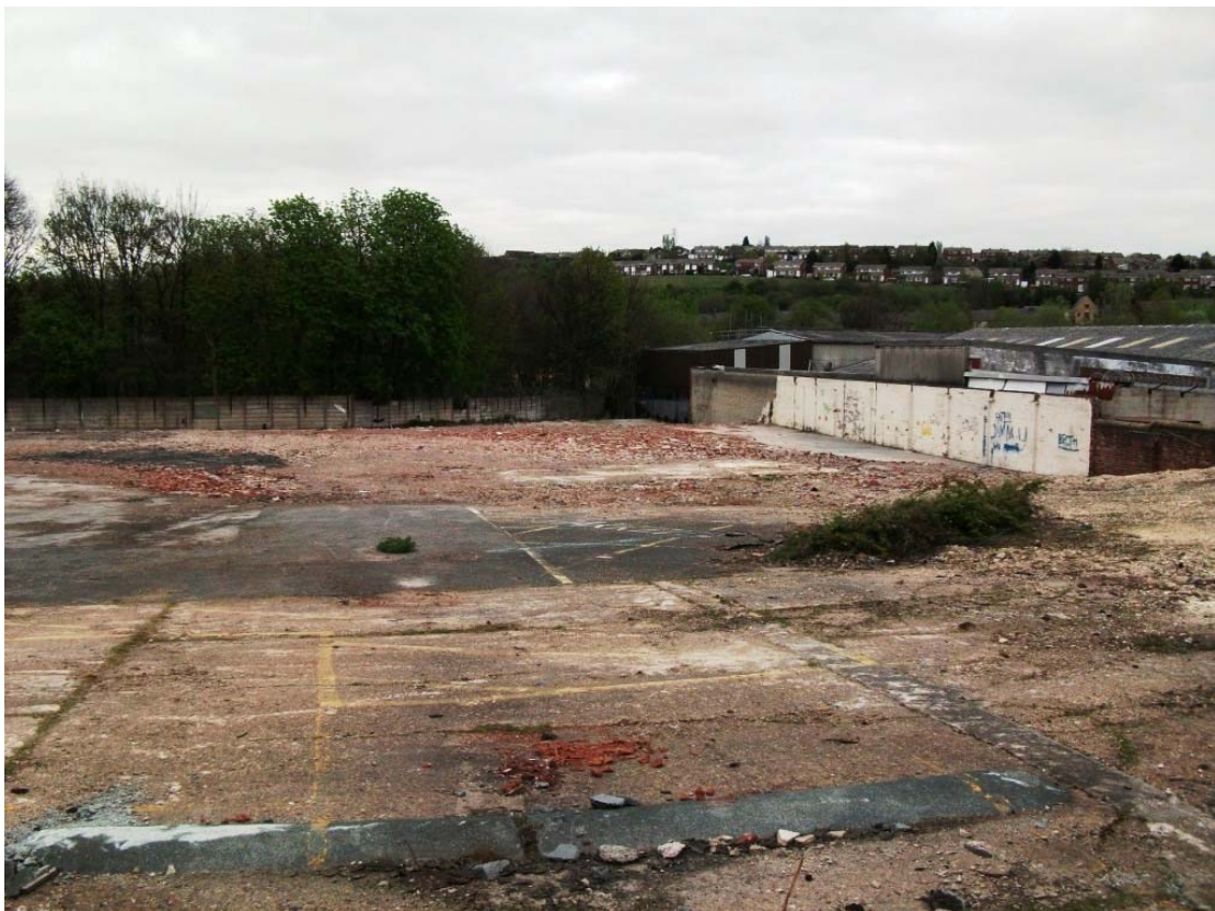
Plate 10: Area of Demolished Buildings, Looking North from Twibell Street
