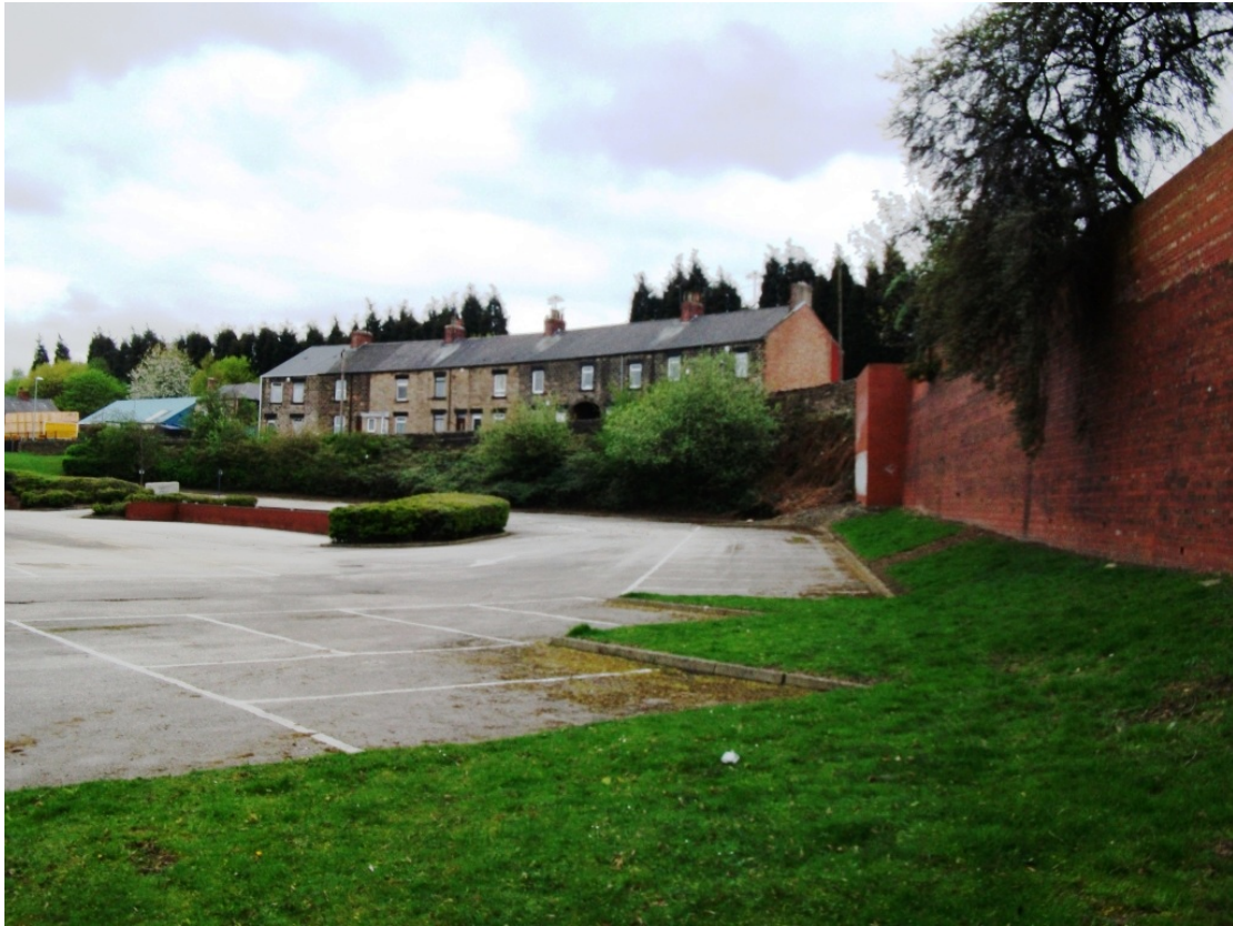
Plate3: Adjacent to the Retaining Wall along Old Mill Lane, towards Twibell Lane
