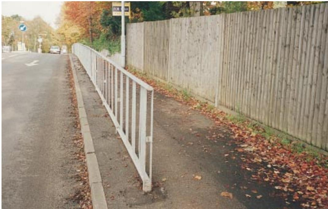
Excessive and unnecessary amounts of pedestrian guard rail should be avoided.
