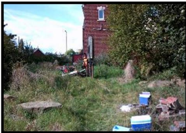
L: Location of window sample borehole WS06
