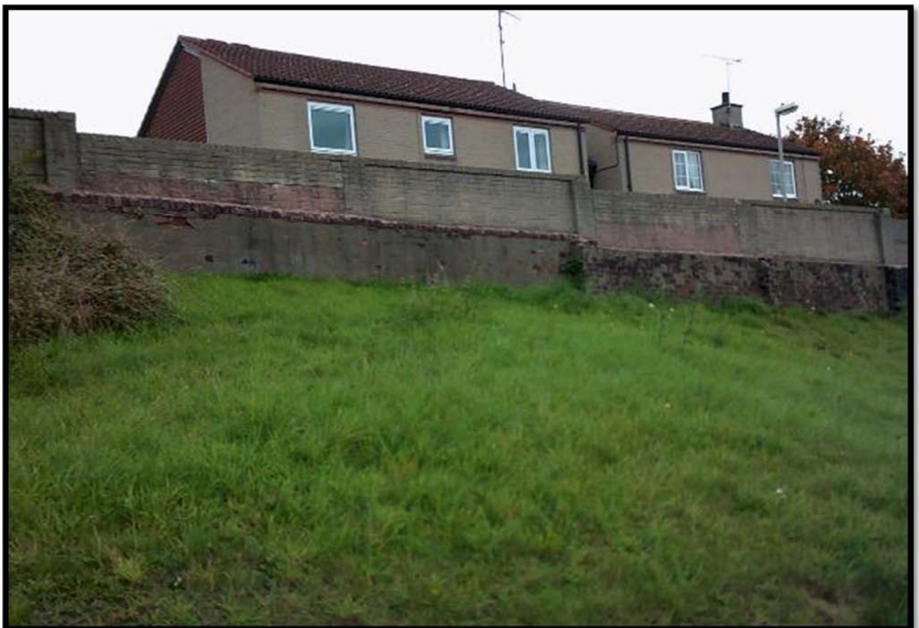
D: The site had been steeply banked at the north boundary.
