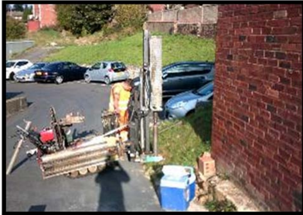
H: Location of window sample borehole WS02
