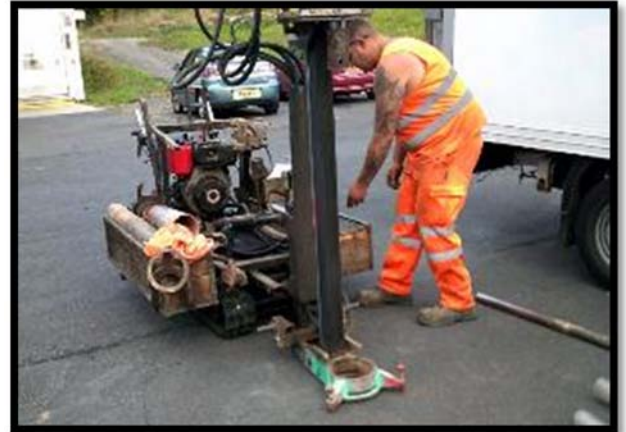
I: Location of window sample borehole WS03
