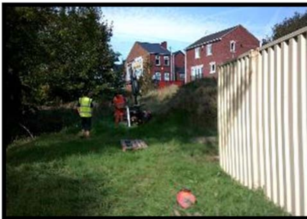
R: Location of window sample borehole WS12
