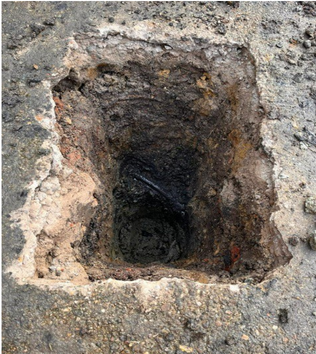
Fig 5 – Pre-drilling Test Pit – Borehole BH1
