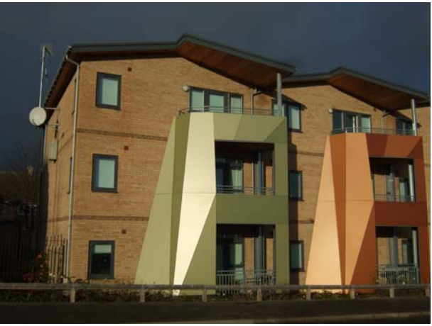
View of the west facade fronting of the apartment complex Pearson Crescent
