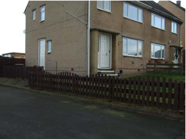
View of two storey housing on the east side of Wortley Avenue opposite Area 2
