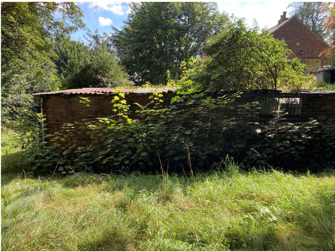
Fig 06. Outbuilding within site built of brick with flat roof.
