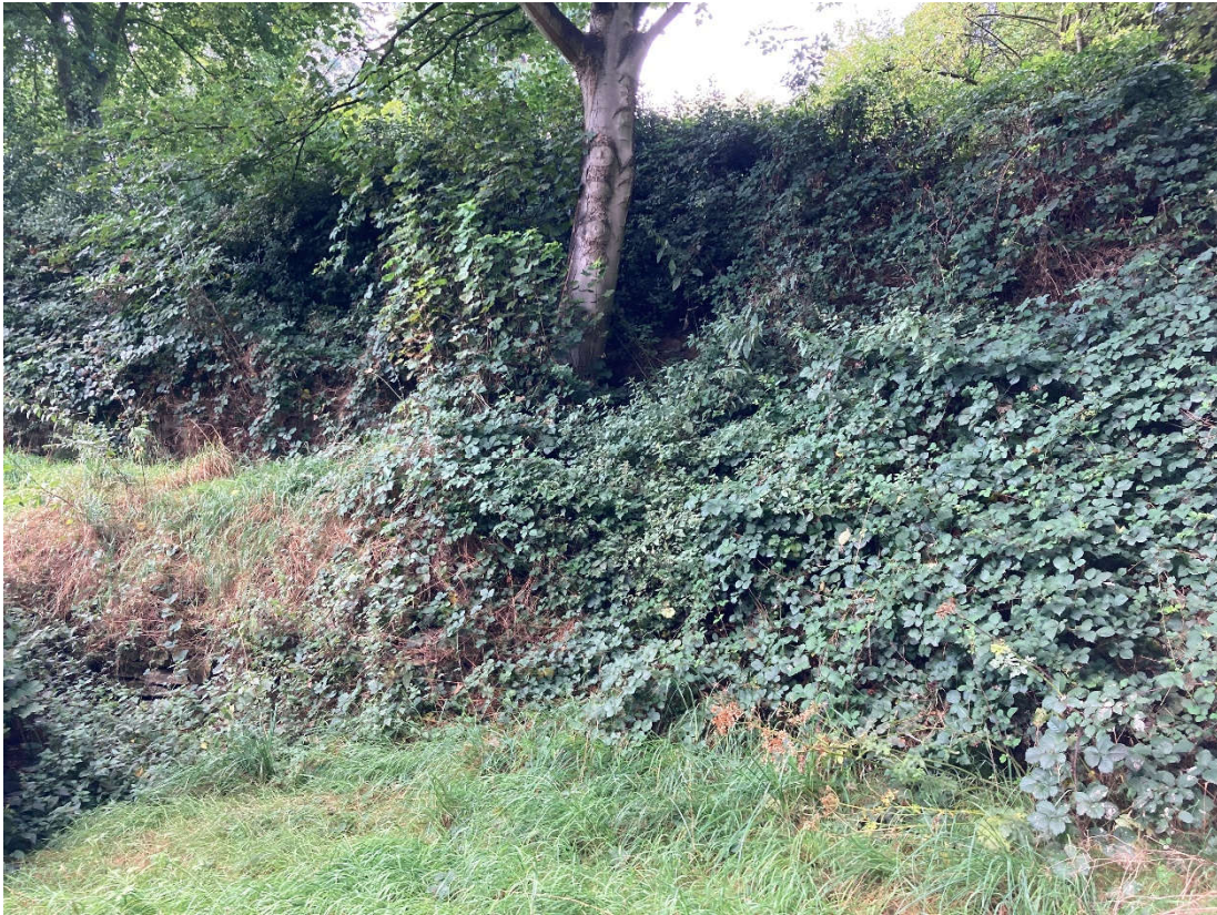
Fig 07. View of T4 above ground level of the site.
