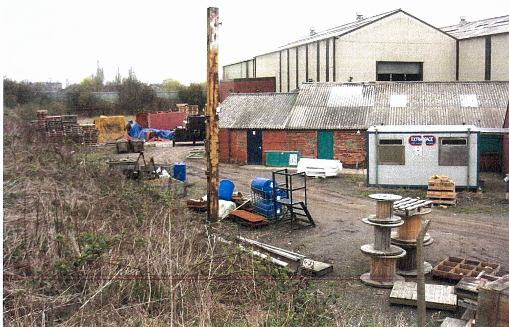
Photograph 6 – View to the east across the site showing the main storage areas and range of buildings.
