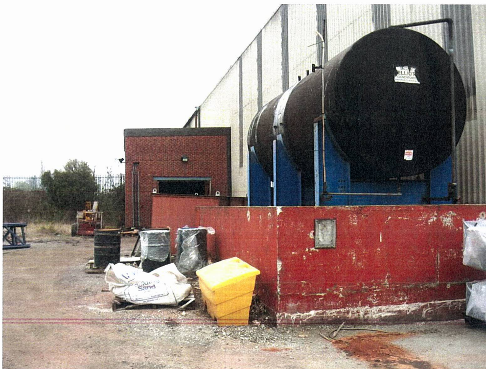
Photograph 4 – Main fuel storage tank, concrete bund in good condition, no evidence of any leaks.
