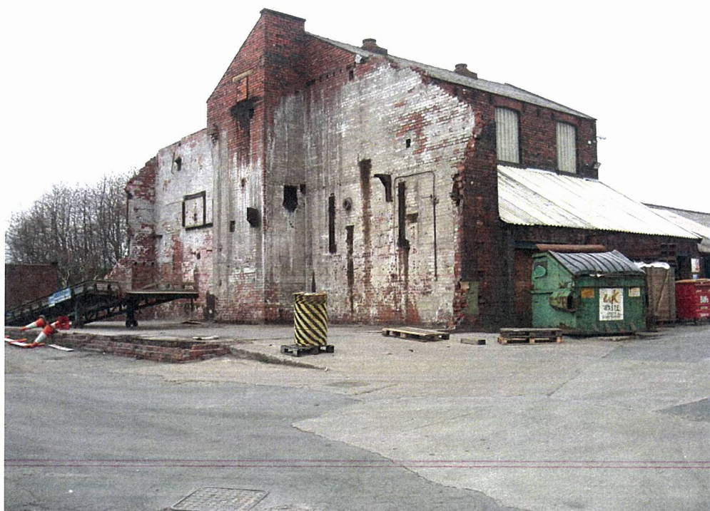
Photograph 8 – View looking northwest towards the part demolished building. Hard stand is noted as in good condition.
