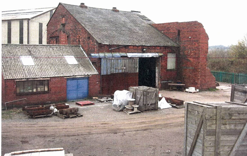
Photograph 7 – Part demolished building to the south of the site.
