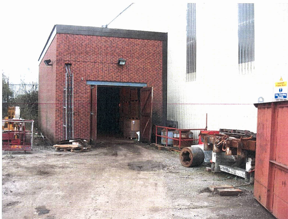
Photograph 3 – View of the proposed development area. Hard stand to the fore of the photograph in good condition.
