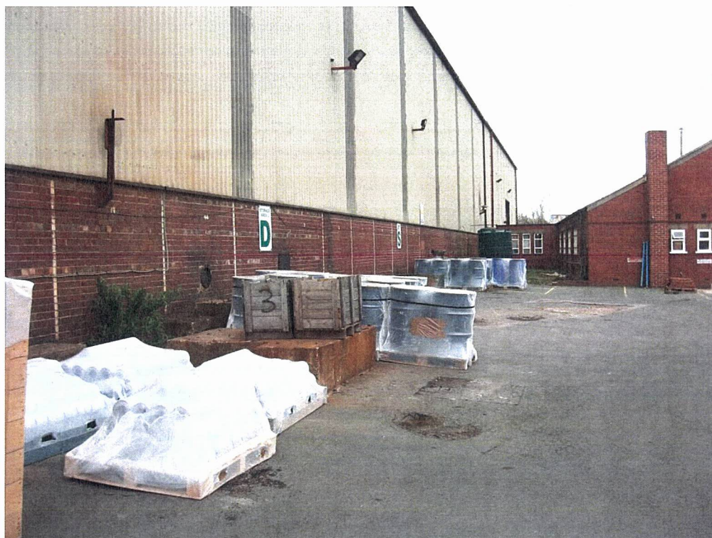
Photograph 9 – View of sites southern boundary following delivery of processing materials. Hard stand is noted as in good condition.
