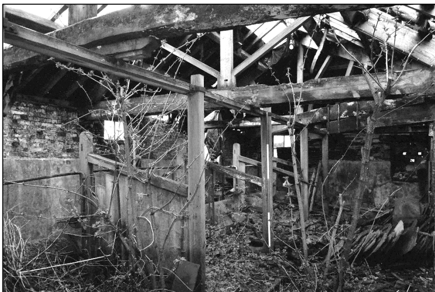
Appendix 2.49: View of the interior of Room GI, Building C , looking north
