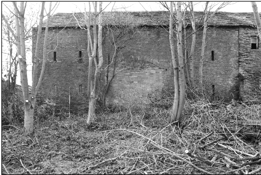
Appendix 2.52: View of the north elevation of Building D looking south
