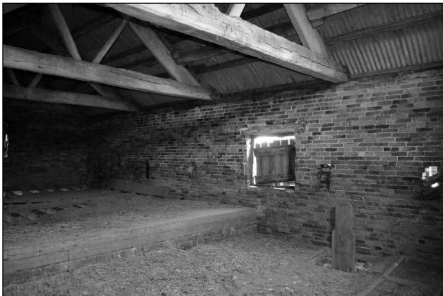
Appendix 2.44: View of the interior of Room FI, Building B , looking south-west
