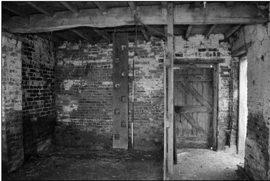
Appendix 2.43: View of the interior of Room G2, Building B , looking west – note jacob's ladder
