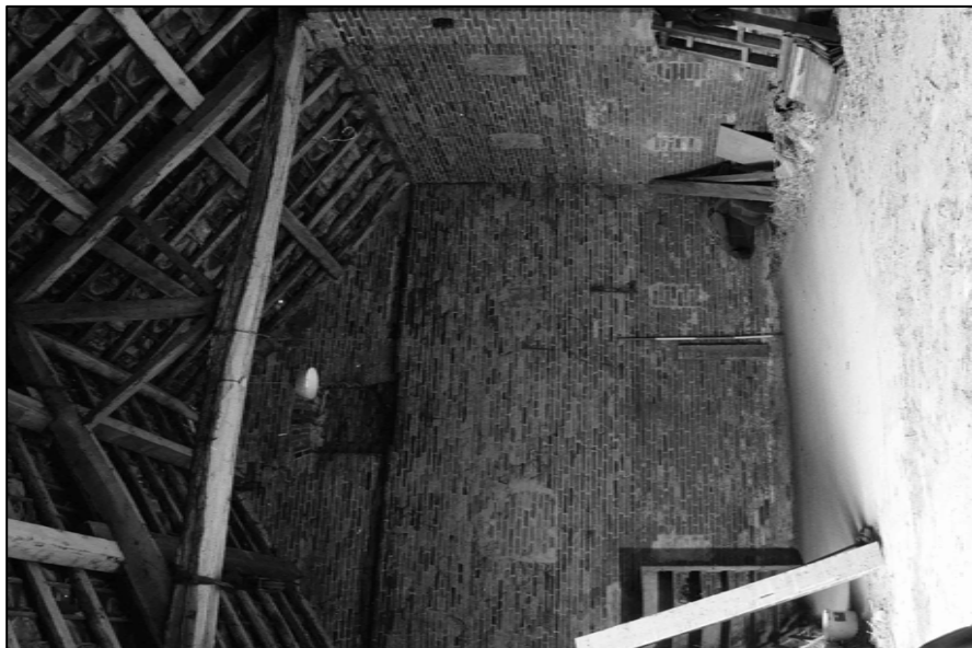
Appendix 2.55: View of the interior of Room G1, Building D, looking west
