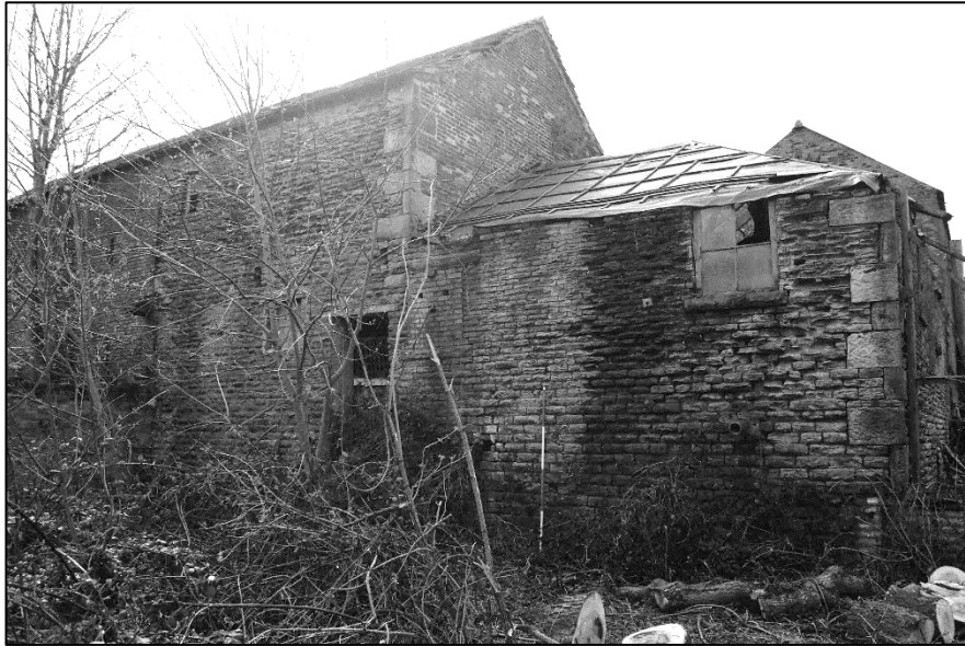
Appendix 2.47: View of the north elevations of Building C and the west bay of Building B looking south
