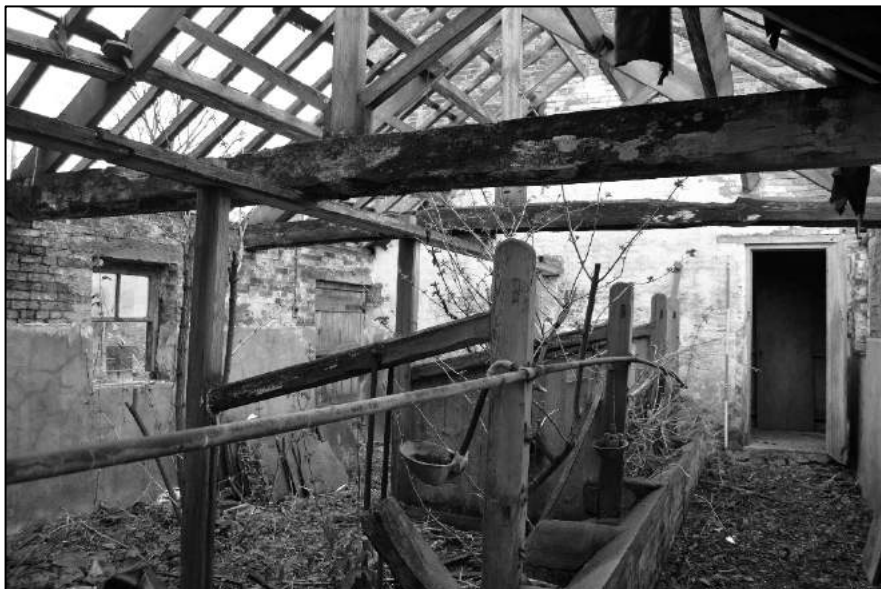
Appendix 2.48: View of the interior of Room GI, Building C , looking south
