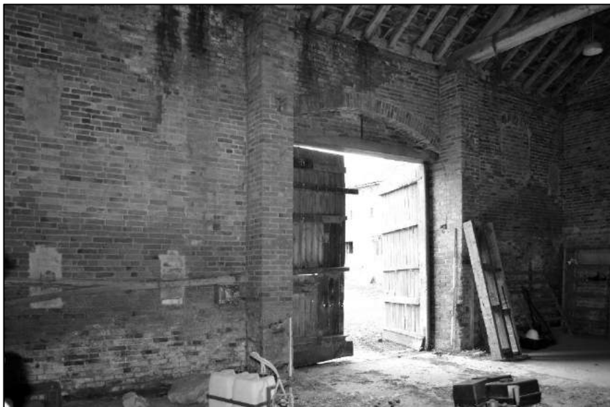
Appendix 2.58: View of the interior of Room G2, Building D , looking south-west
