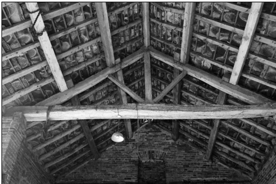
Appendix 2.61: View of the west roof truss above Room G2, Building D, looking west
