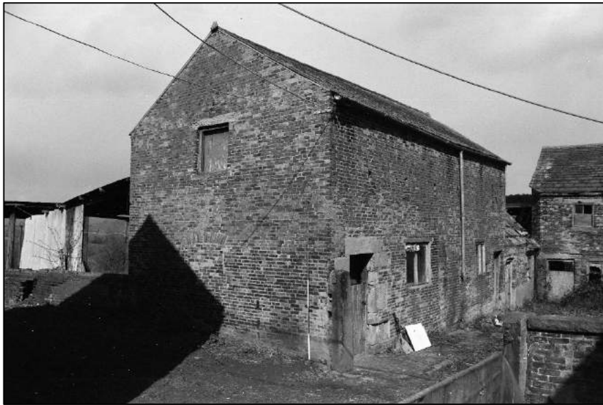
Appendix 2.40: View of the south and east elevations of Building B looking north-west
