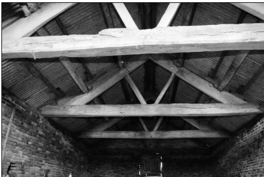
Appendix 2.45: View of the roof trusses above Room FI, Building B , looking south
