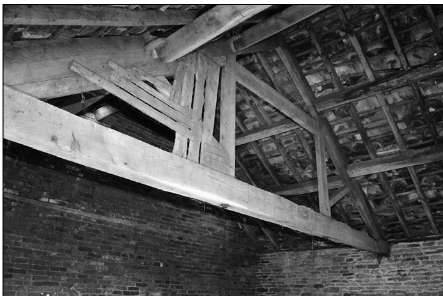
Appendix 2.62: View of truss above Room FI, Building D, looking
