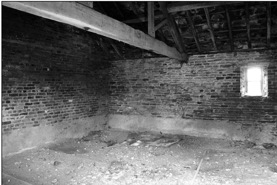
Appendix 2.60: View of the interior of Room FI, Building D, looking north-west
