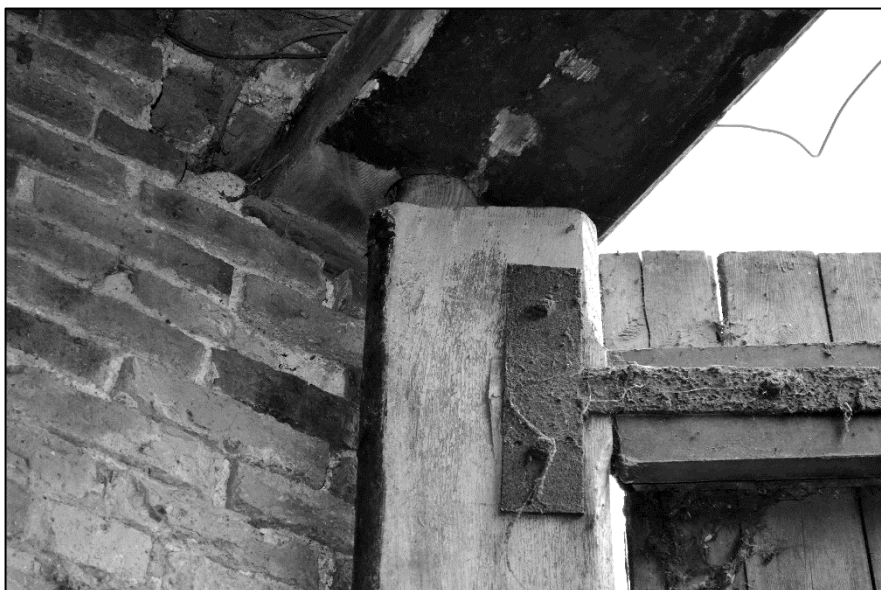
Appendix 2.59: Detail of hammer-hung hinge of door in south elevation of Room G2, Building D , looking south-east
