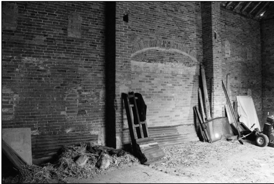
Appendix 2.57: View of the interior of Room G2, Building D , looking north-east. Note central blocked doorway.
