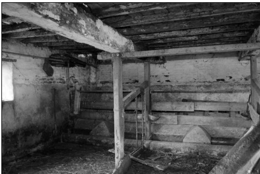
Appendix 2.54: View of the interior of Room G1, Building D , looking east
