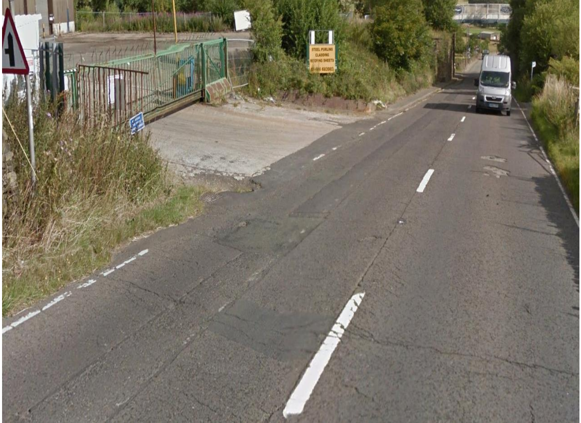
Manchester Road at the Existing Site Entrance
