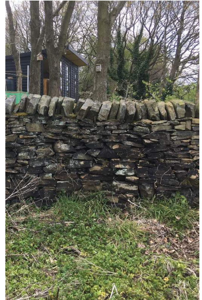
Natural dry-stone wall (site boundary)
